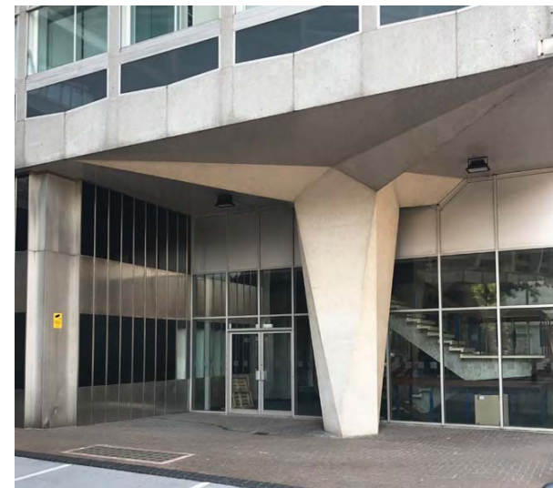
Existing view of Kingsway south stair
