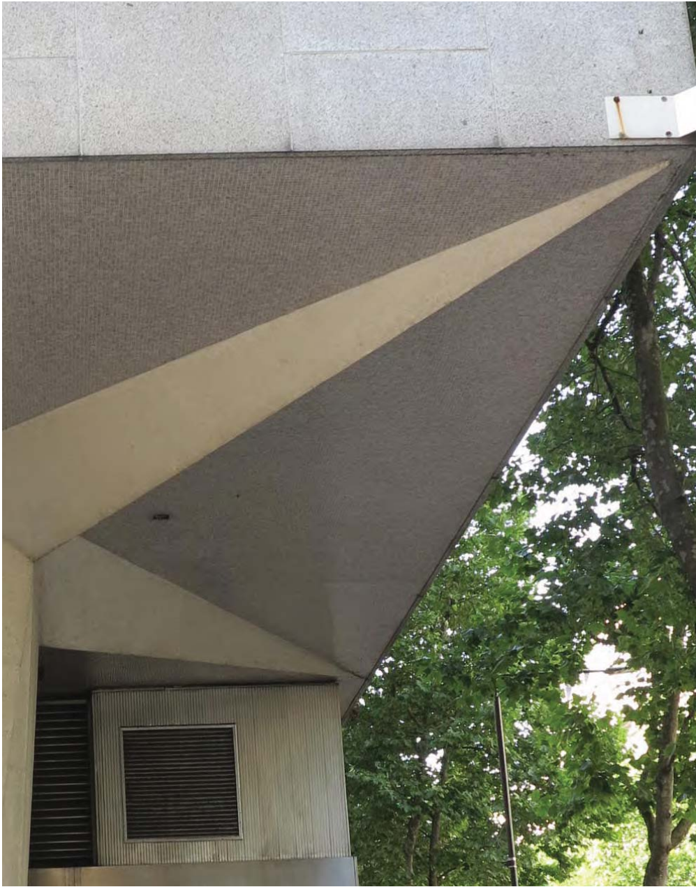
Existing view of mosaic tiled soffit
