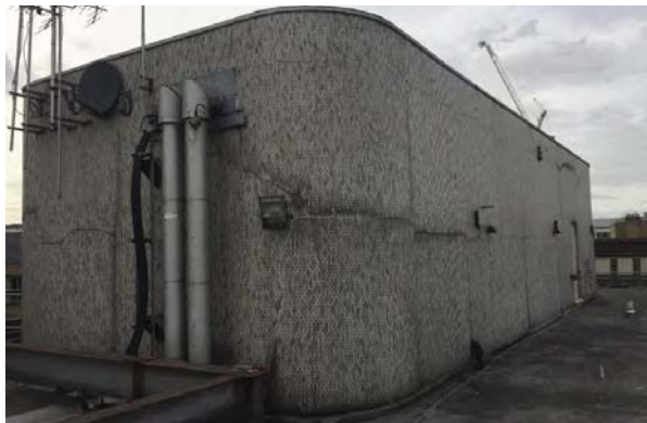
Existing MosaicTiled Plant Room to Kingsway
