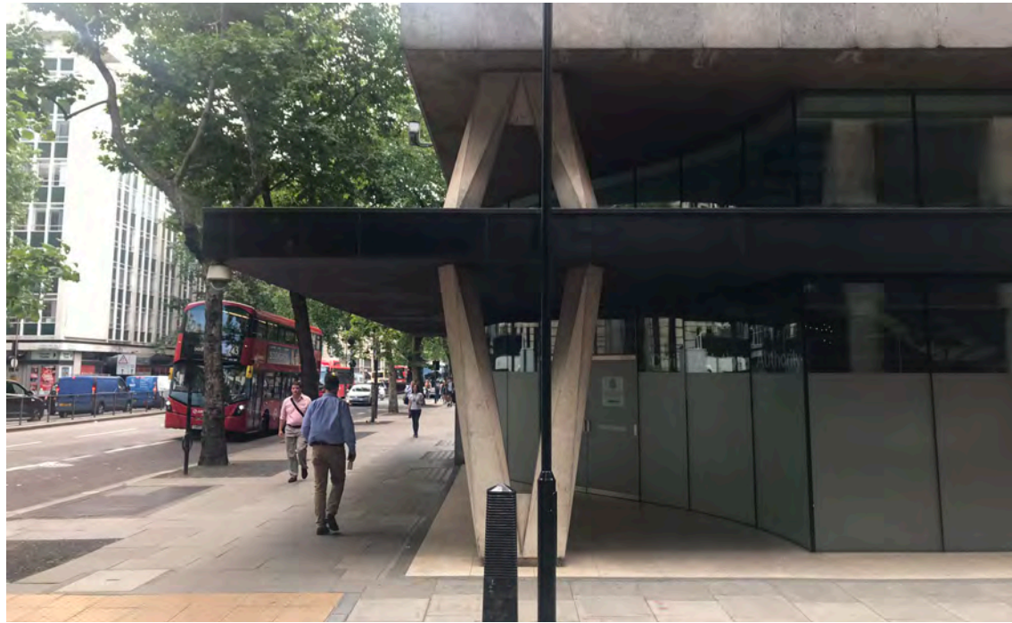
Existing view of Kingsway Northern corner
