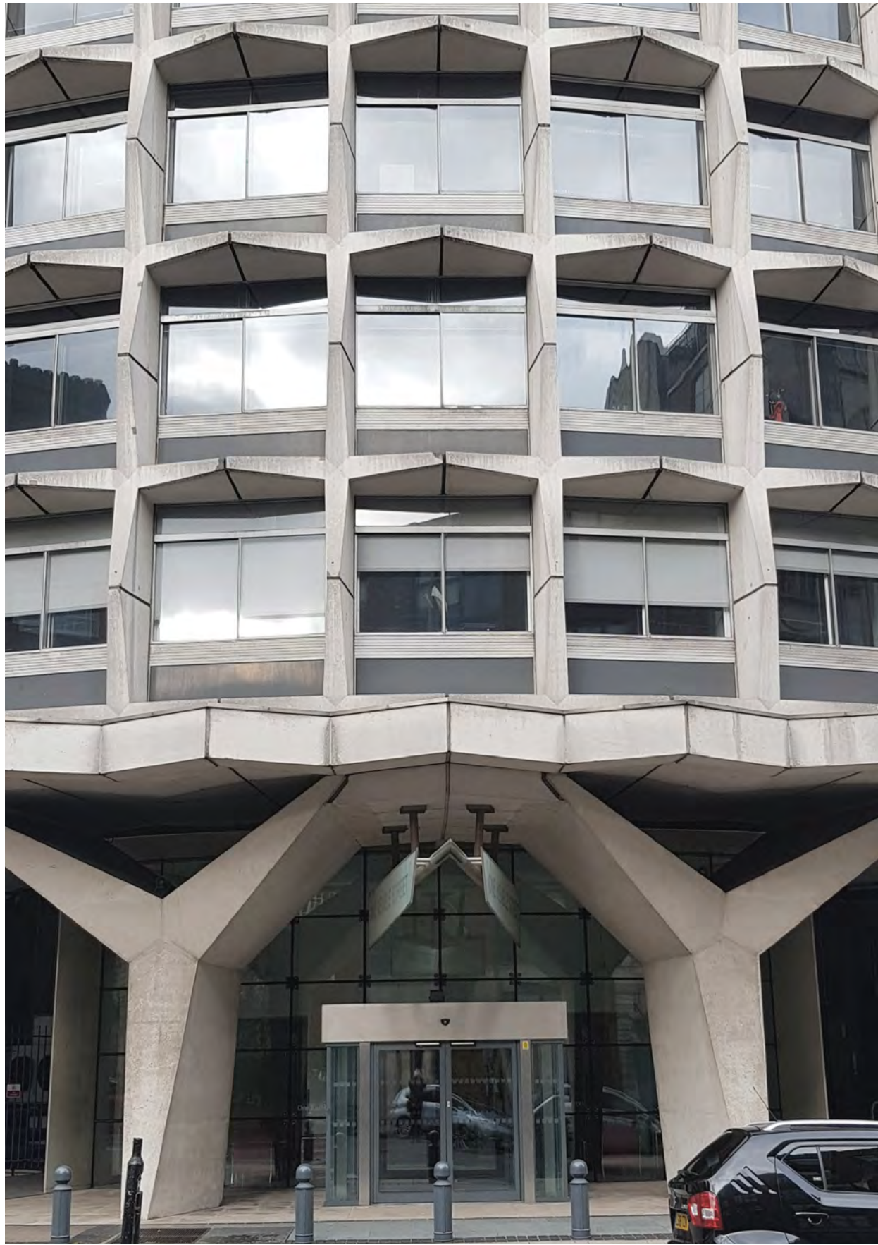
Existing view of tower entrance
