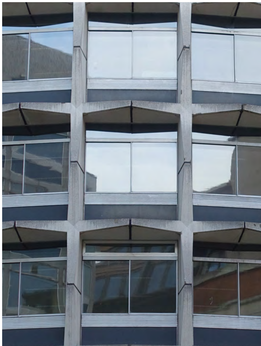
Space House - Existing Photograph
