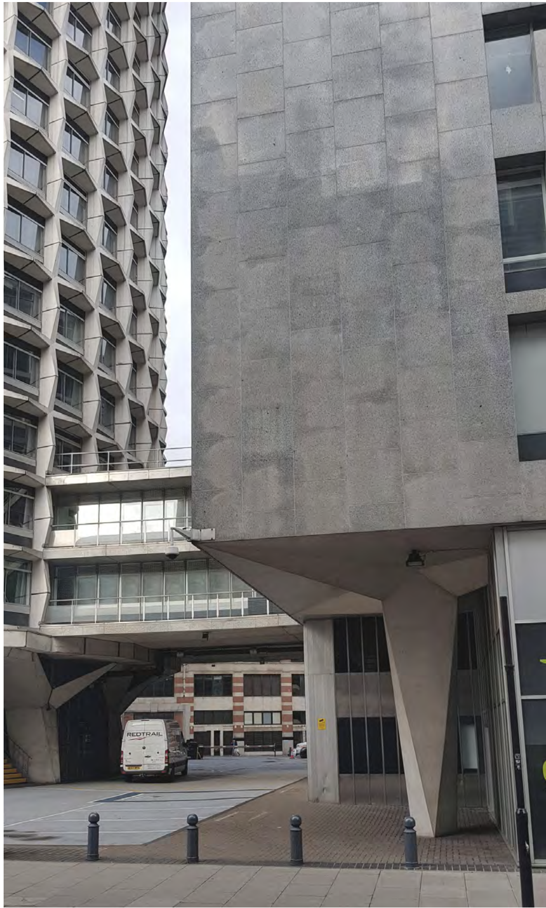
Existing of Kingsway south stair
