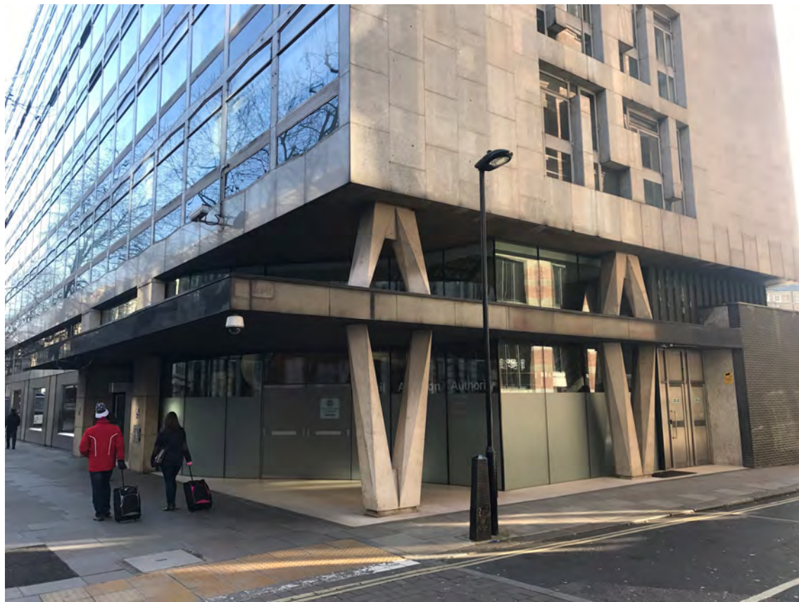
Existing view of Kingsway Northern corner
