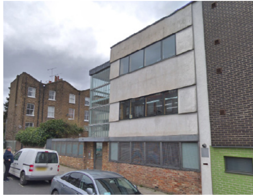
2. Neighbouring No.113 Bartholomew Road.
