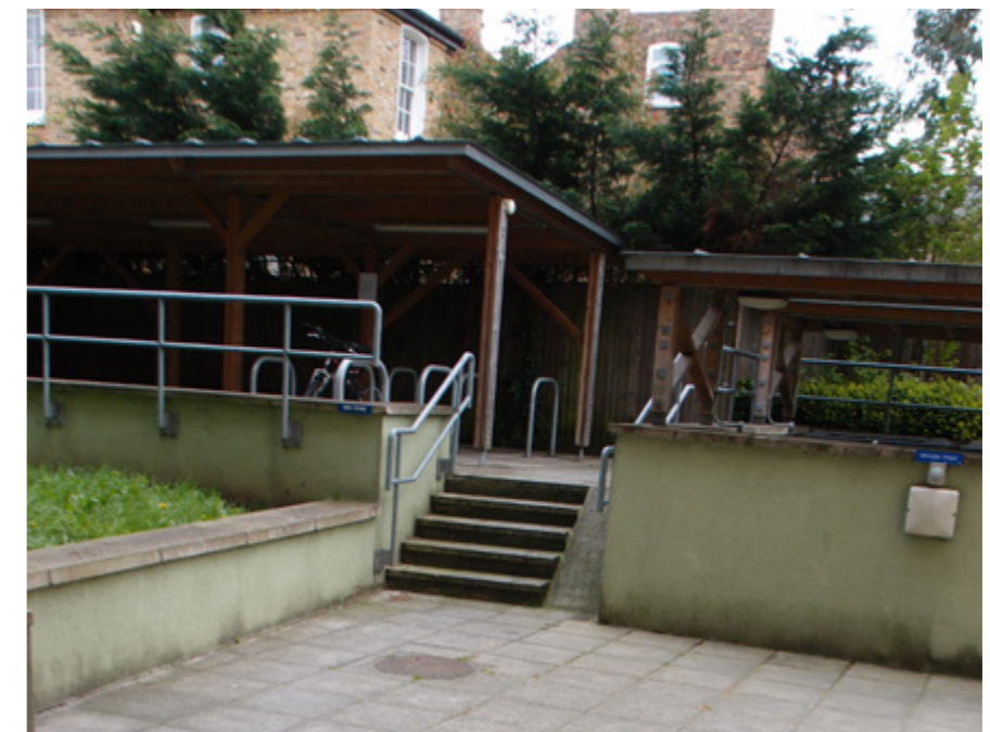
6. Covered cycle storage in rear external space. Dwellings on Torriano Cottages to the rear of the site shown.
