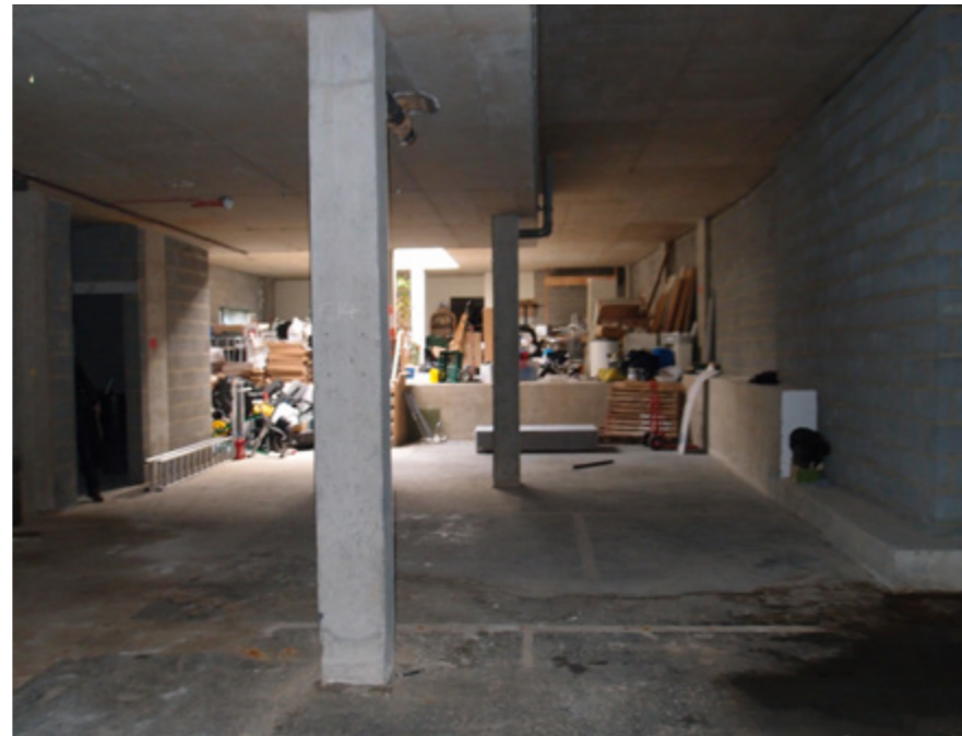
8. Interior view of commercial unit facing towards rear of site.
