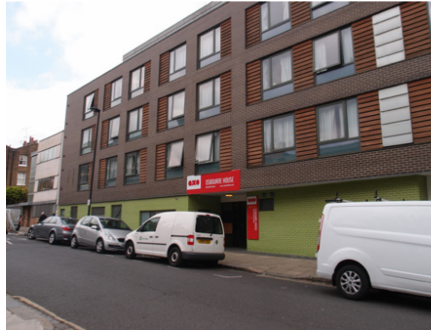
1. View of front (west) elevation of Osbourne House Bartholomew Road
