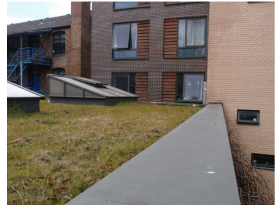
3. View of green roof over commercial unit and rear (east) of student accommodation.
