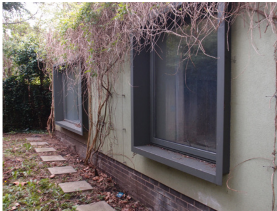
4. View of north facade of commercial unit, overlooking rear external space.
