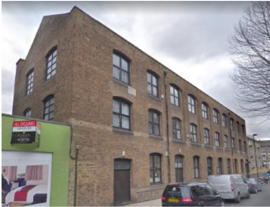
1. Neighbouring No.109 Bartholomew Road.
