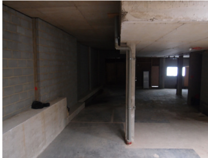
7. Interior of commercial unit facing toward Bartholomew Road.
