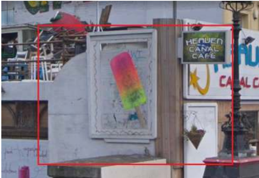
Fig 1. Existing Timber Structure over Canal Bridge Wall by which the roof is currently being accessed– Side view
