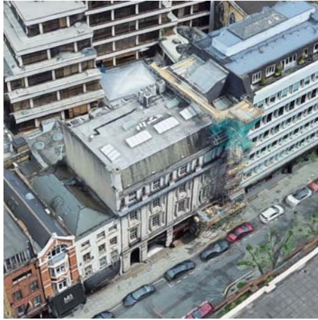
This aerial image shows the building from the front.
