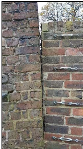
Photo 4: Open joint between pier and wall
