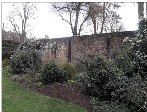
Photo 3: Steel supports securing the boundary wall
