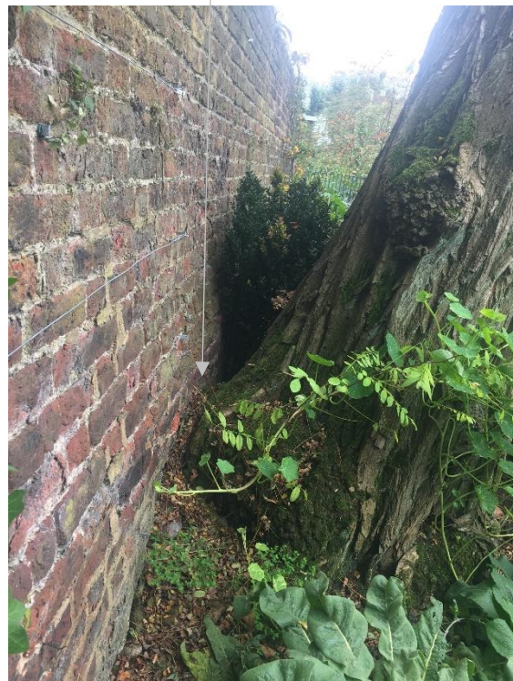
Figure 10 - Robinia pushing inner side of wall
