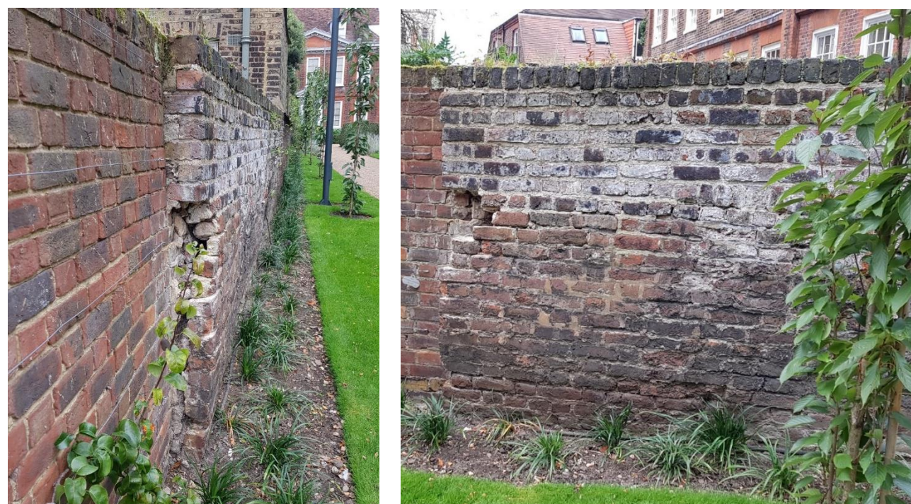
Figure 19 - Opening from delamination of inner skin
