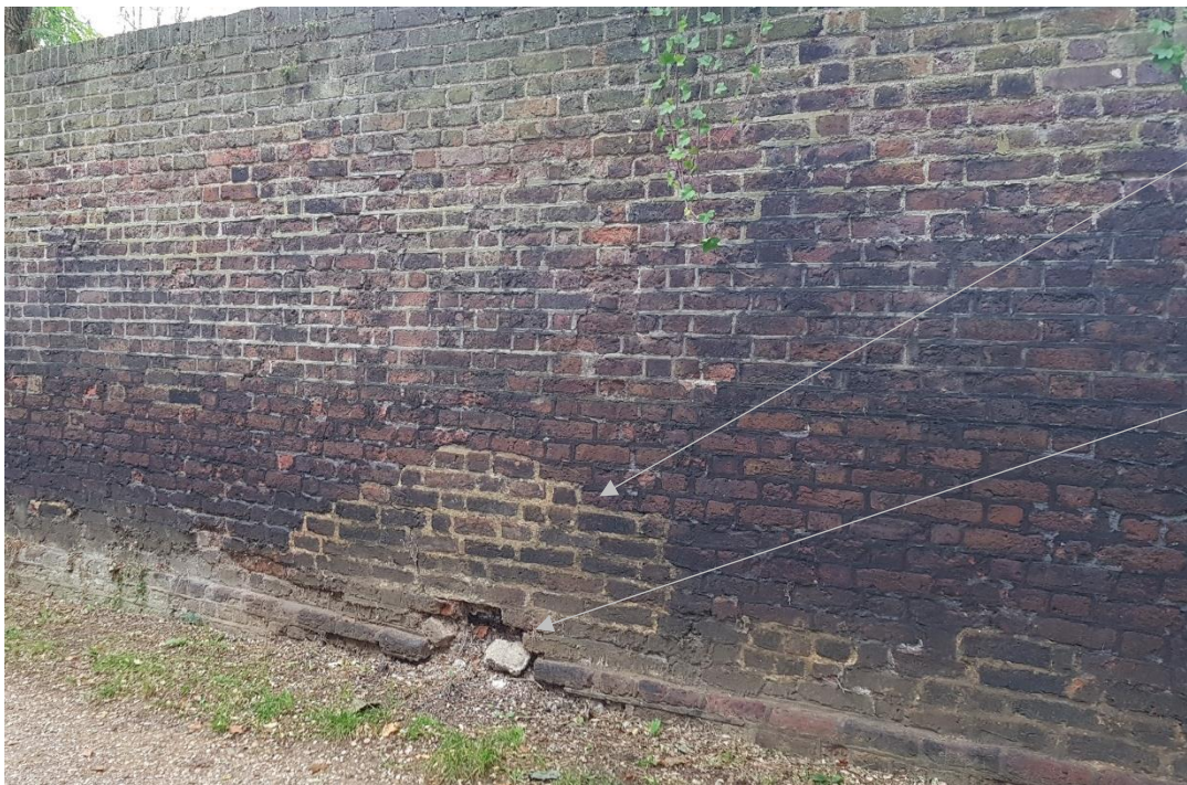
Figure 4 - Local repairs along surveyed section of boundary wall
