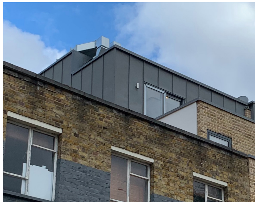
Fig 14. The only bit of the rooftop additions, applied for here, that can be seen from King's Mews is the corner of a duct (seen as shiny here but will be atrhacrite grey)
