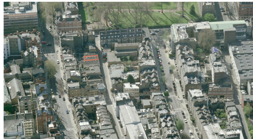
Fig 4. Bird's eye view Looking South - site marked in red
