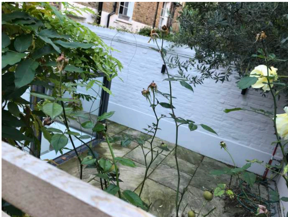
Part view of No. 57 Flask Walk rear extension.
