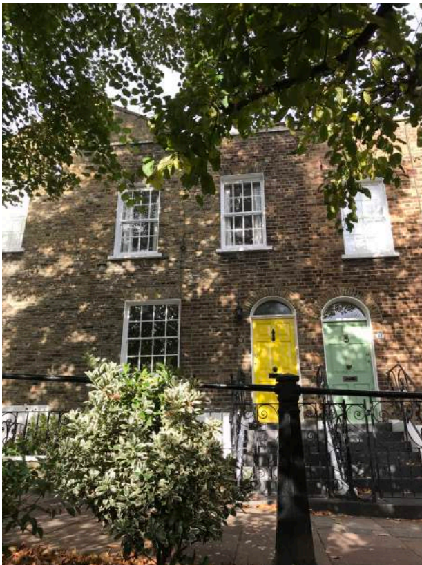
Front elevation – No. 59 with yellow door
