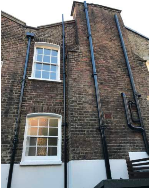
Rear elevation upper
