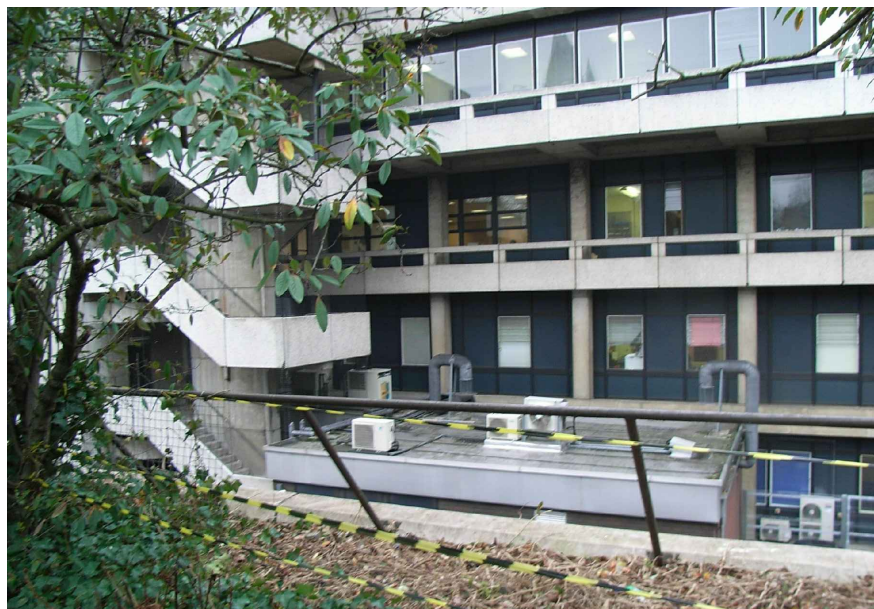
rooftop views of existing MRI 4
