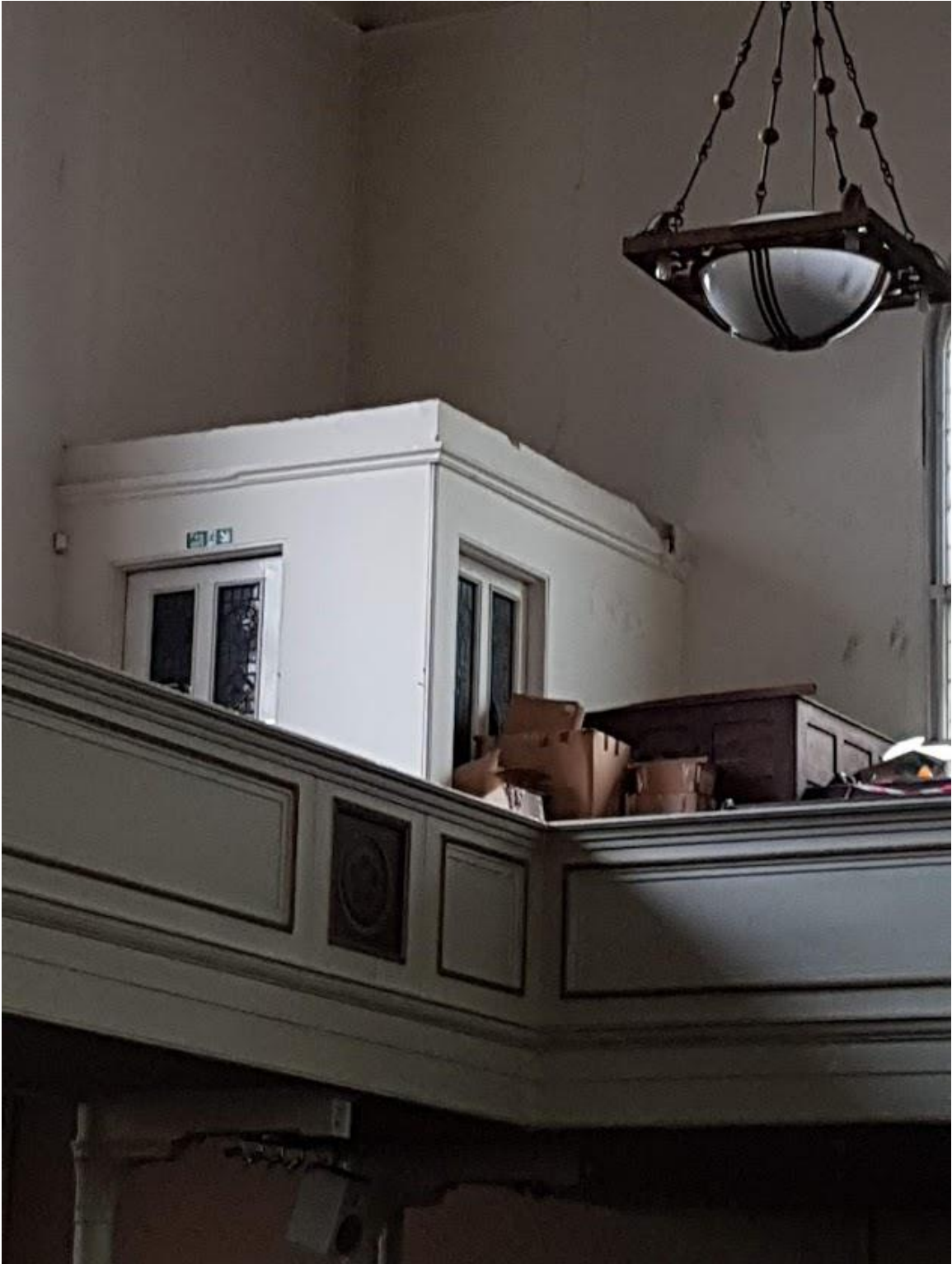
Existing staircase enclosure which we will match.
