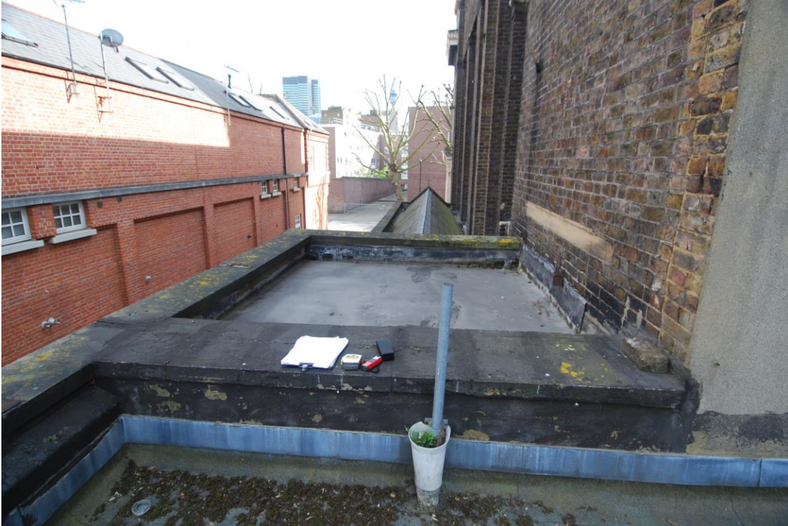
Roof area over the entrance lobby
