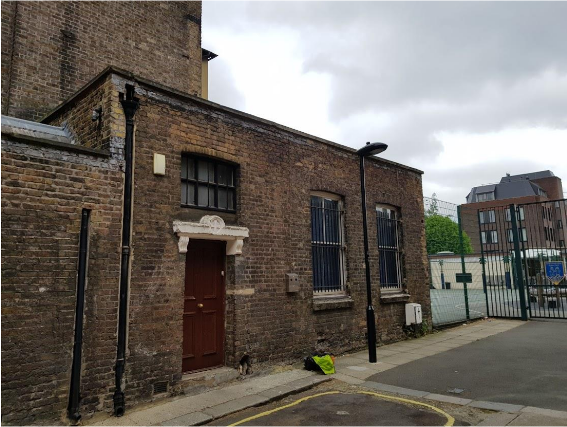
Little Edward Street - Annex building over which the new first floor will be built.
