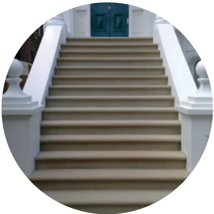
York Stone Steps with bull nose detailing
