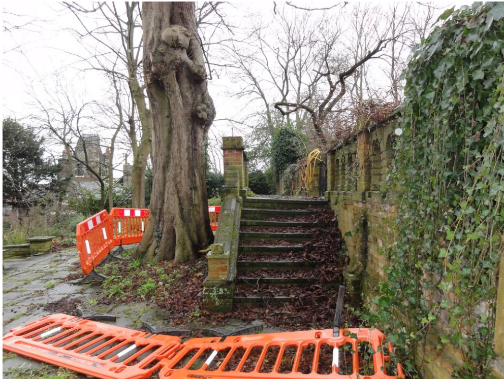
Photograph 3 – Side elevation of stairs and tree.
