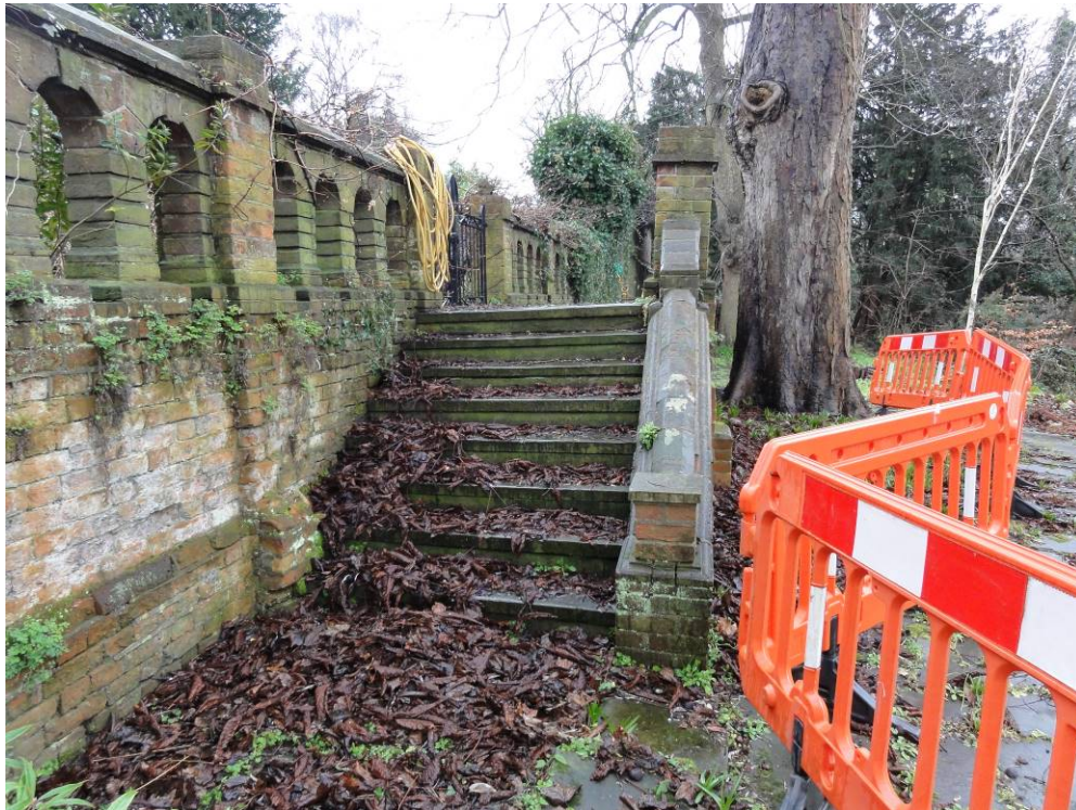
Photograph 7 – Side elevation of stairs and tree.
