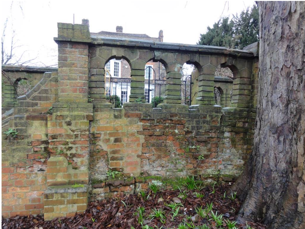
Photograph 1 – Front elevation of wall, balustrade and tree.
