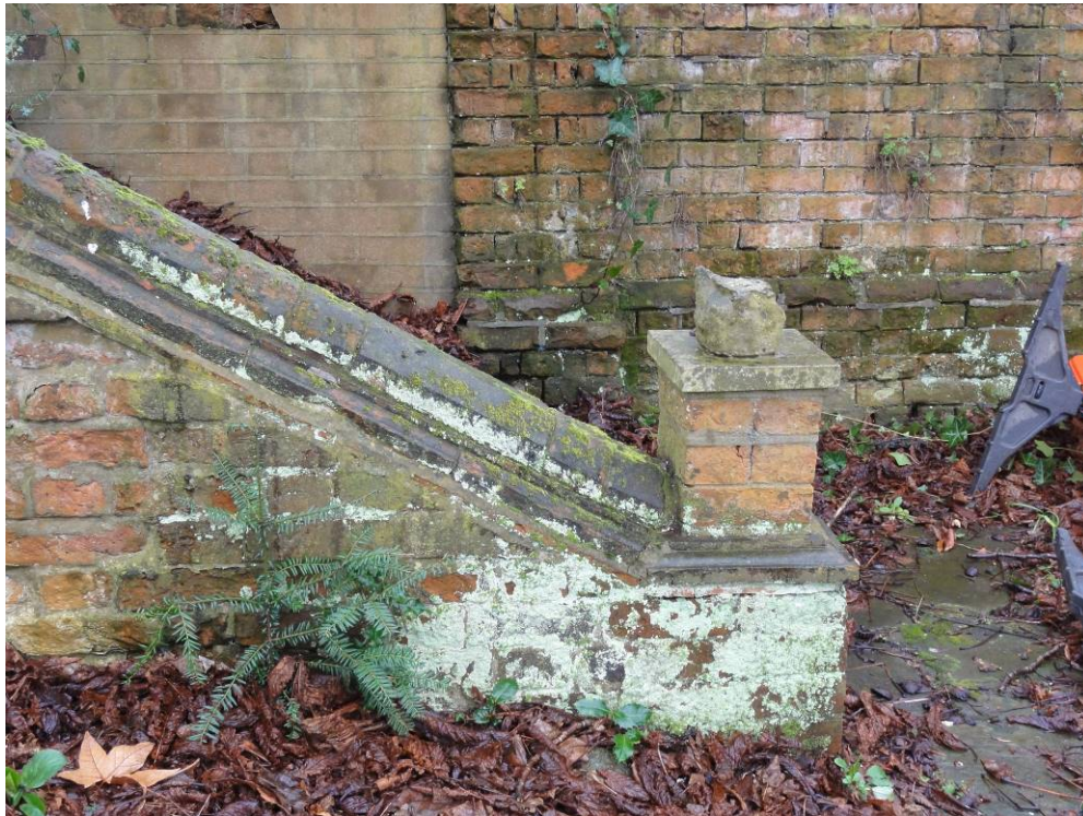
Photograph 5 – Lower section of stairs.
