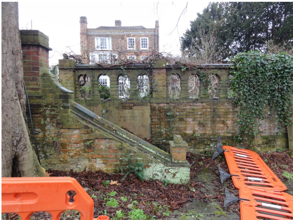
Photograph 2 – Side elevation of stairs and tree.
