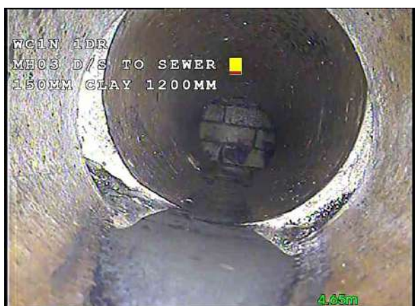
MH03X_db4c3902-a805-424c-9d19-91b8378396aa_20180520_171714_316.jpg, 00:00:42, 4.65 m Joint displaced, large
