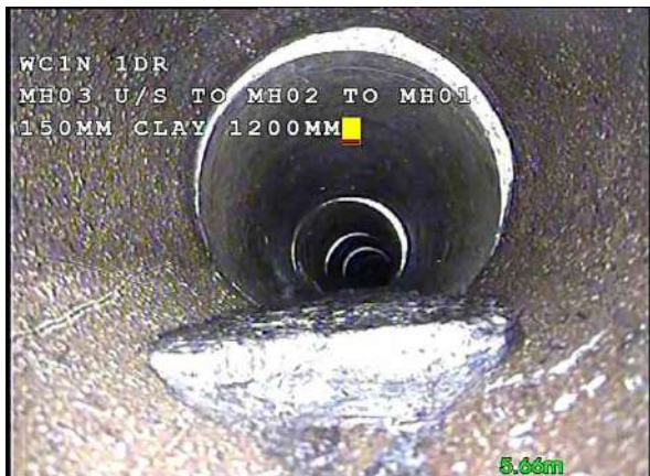
MH01X_cf1ed632-094b-4c90-9aed-09c6bcffc7b1_20180520_170938_300.jpg, 00:01:05, 5.66 m Settled deposits, hard or compacted, 5% cross-sectional area
