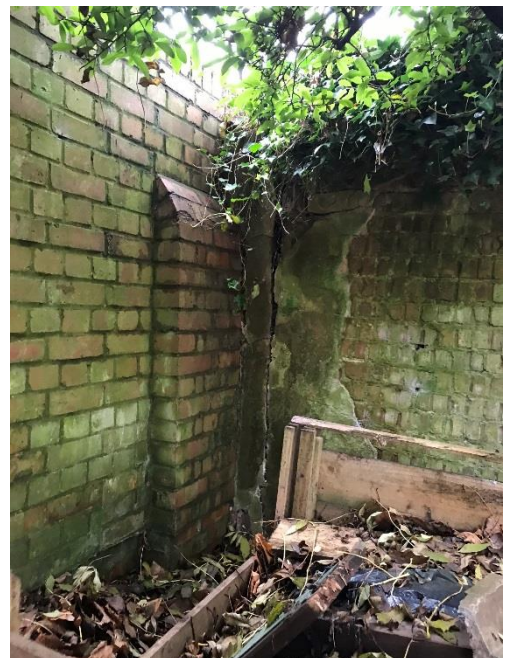
8. Buttress 5 & left hand side wall of oil store. Note crack in oil store wall.
