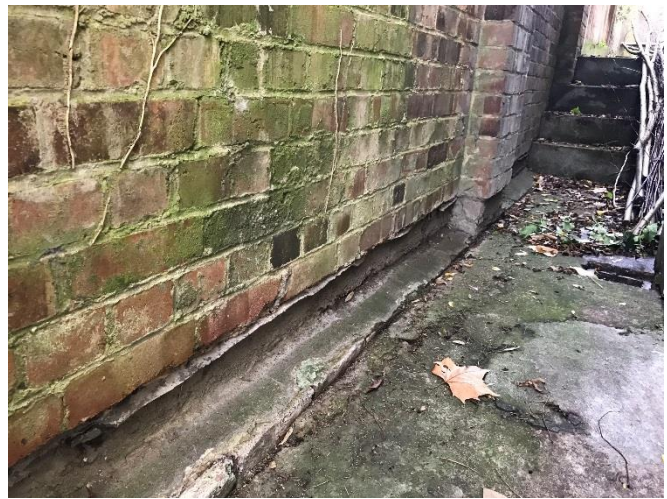
26. Low level of wall panel 10, note lateral movement above DPC.
