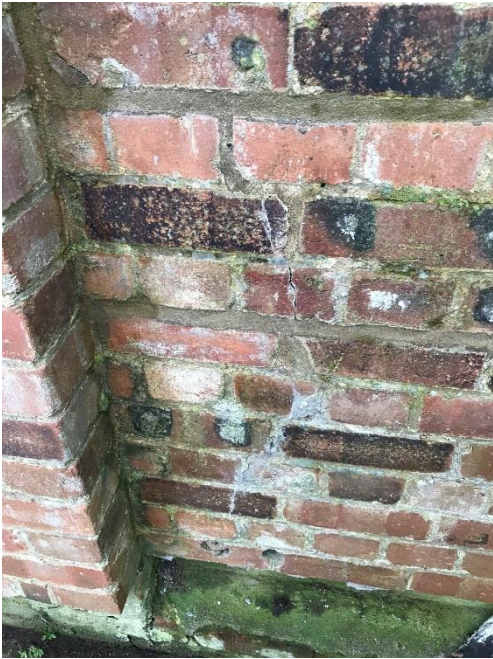
25. Low level of wall panel 10, note weep hole.
