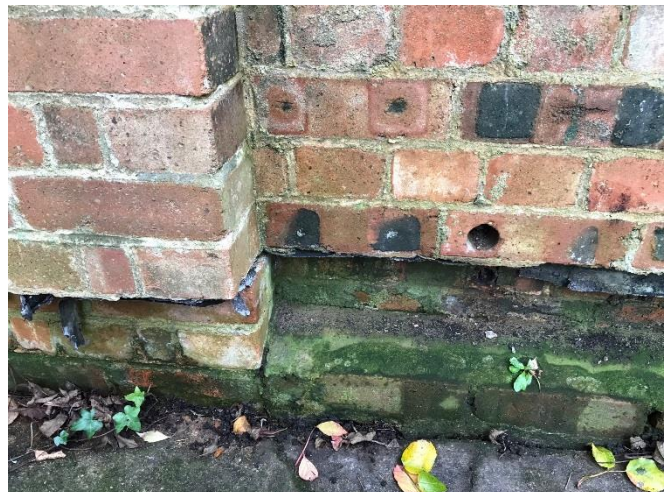
20. Low level of wall panel 9, note weep hole and lateral movement of wall.
