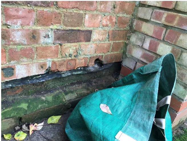
21. Low level of wall panel 8 and buttress 9, note weep hole. It would appear there has been no lateral movement since buttress 9 has been constructed.
