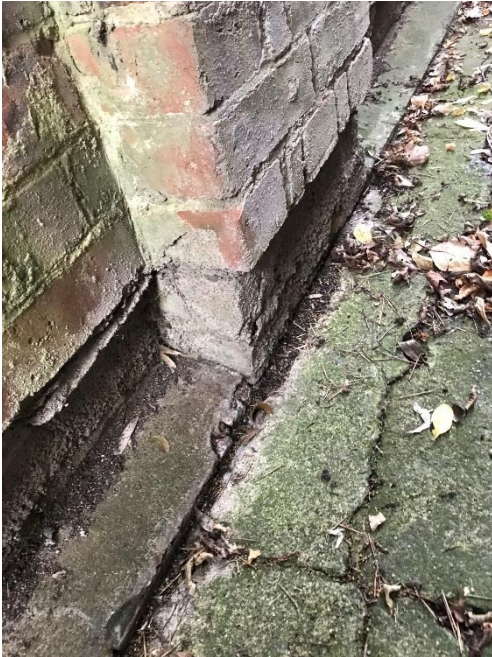
29. Low level of buttress 11, note historic lateral movement above DPC.
