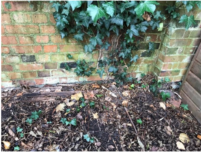
13. Low level of wall panel 6. Note wall moved laterally.
