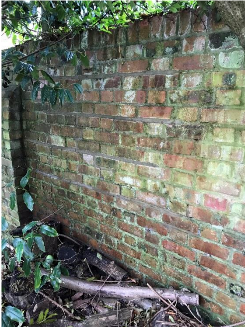
5. Panel 4. Note previous Helibar remedial repairs and poor condition of mortar bottom 6 courses.
