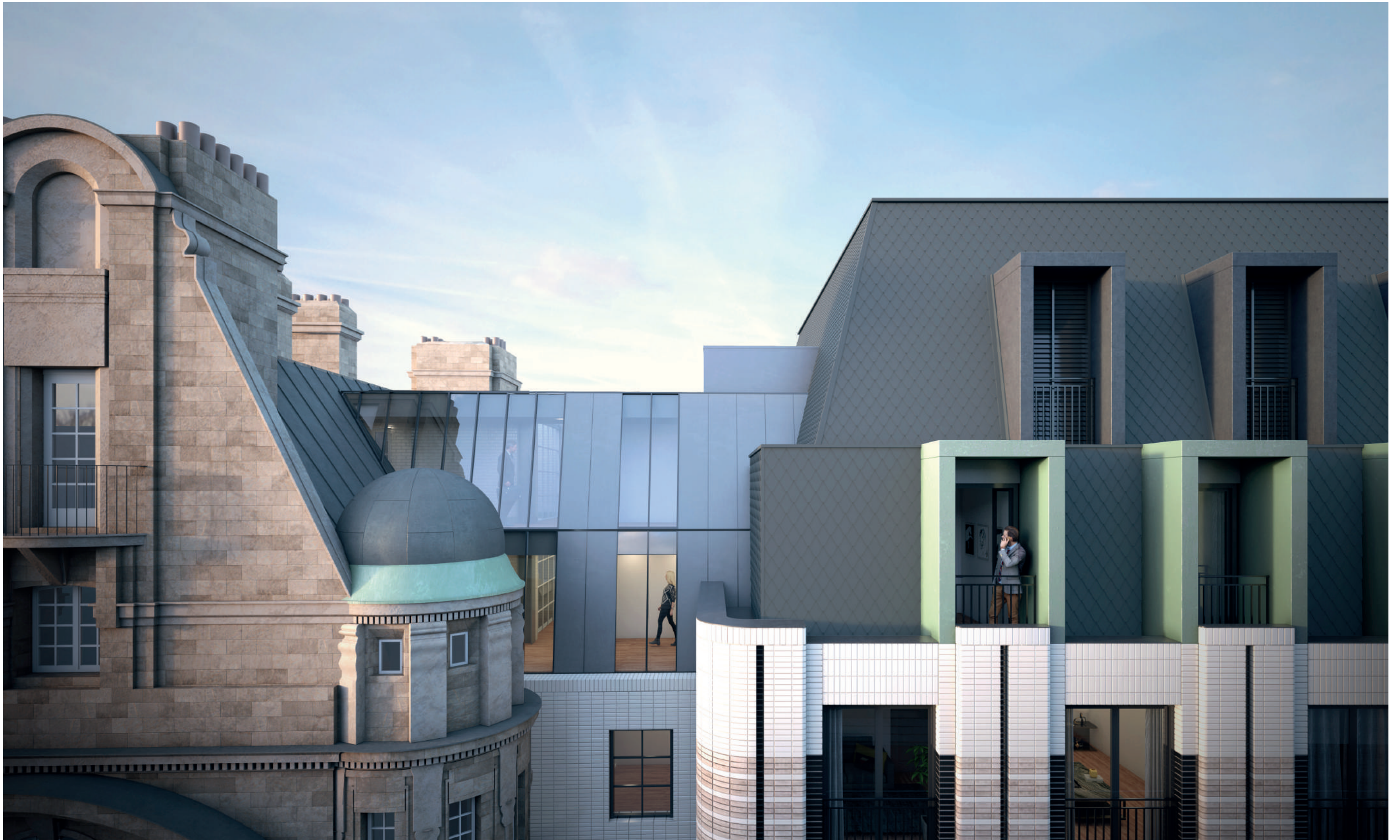
CGI showing new glazed link at 6th & 7th floor. The mansard roof shape reveals the maximum possible area of the existing 'catslide' roof and mediates between old and new.
