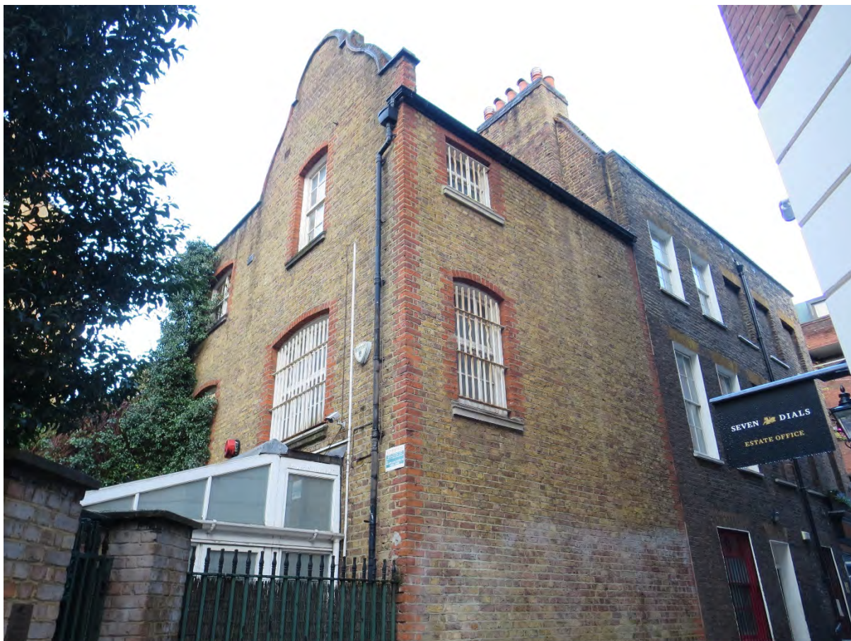
Image EDP 1: 2 Tower Court, looking north-west.
