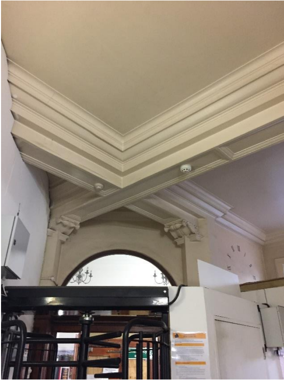
Plate 2: Ground Floor ceiling with replica down stand cornices
