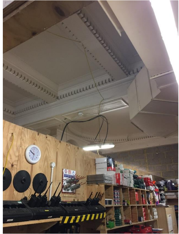
Plate 5: Ground Floor ceiling with replica down stand cornices
