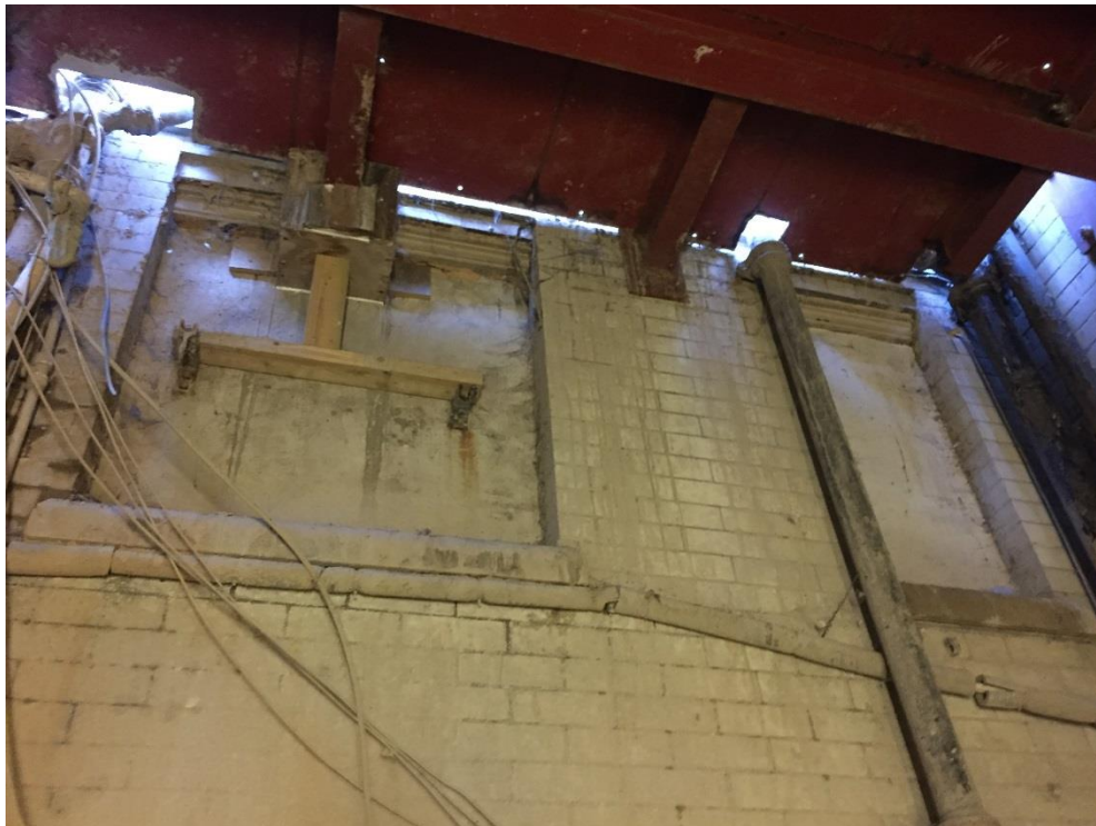
Plate 3: Remnant of rear elevation within lightwell at lower ground floor level
