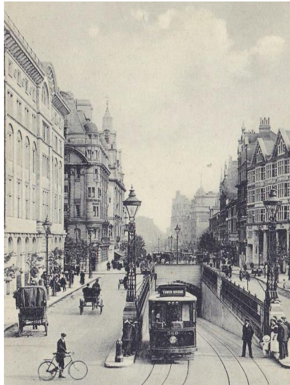
Plate 10: Edwardian photograph of Southampton Row looking south
