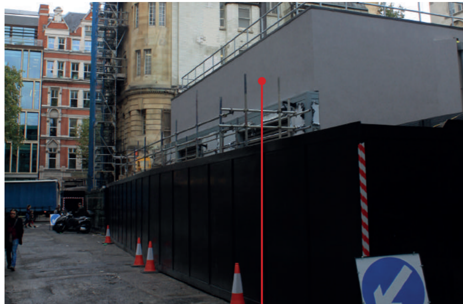
TfL Headhouse now completed
