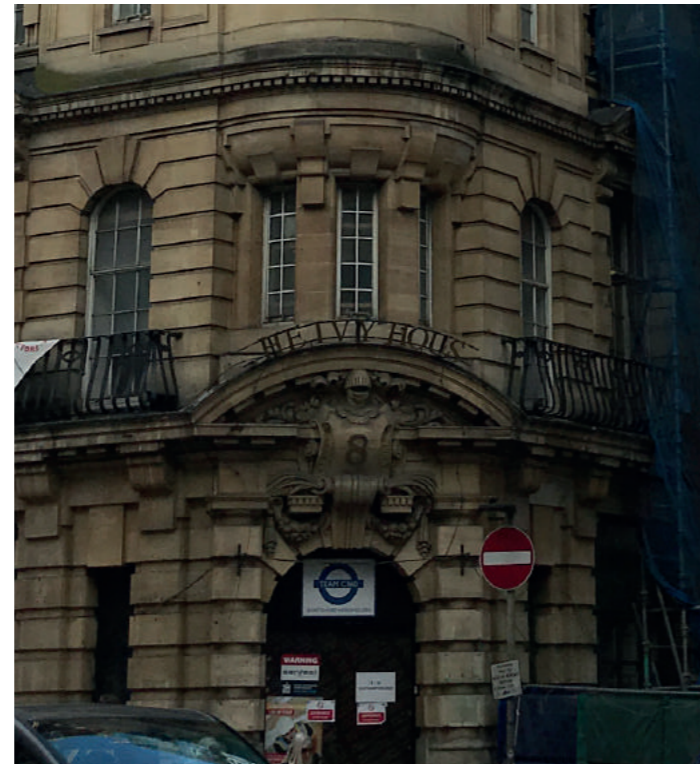
Carlisle House - decorative southwest entrance and first floor balustrades
