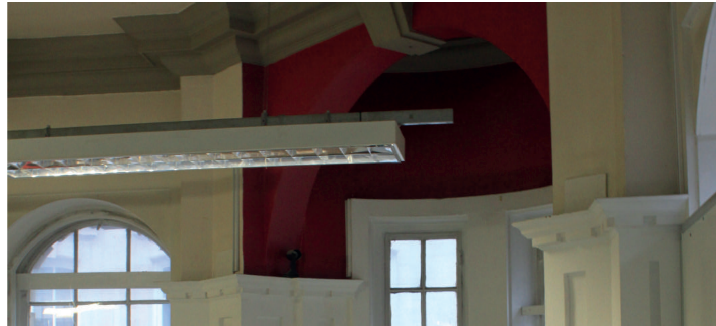
Decorative cornices & beams at 1st floor ceiling
