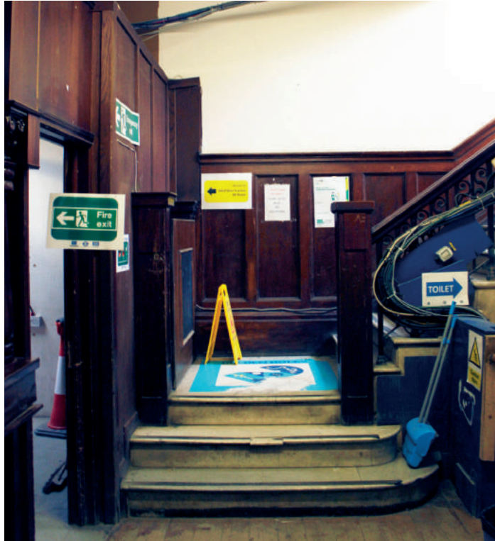
Ground floor stair & 1996 Edwardian style joinery to the left
