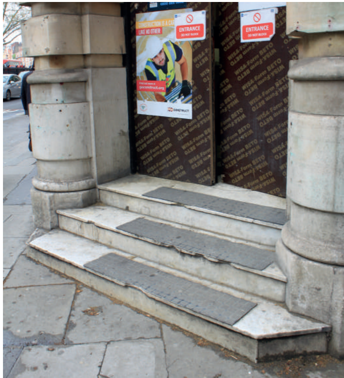
Carlisle House - stepped entrance at southwest corner
