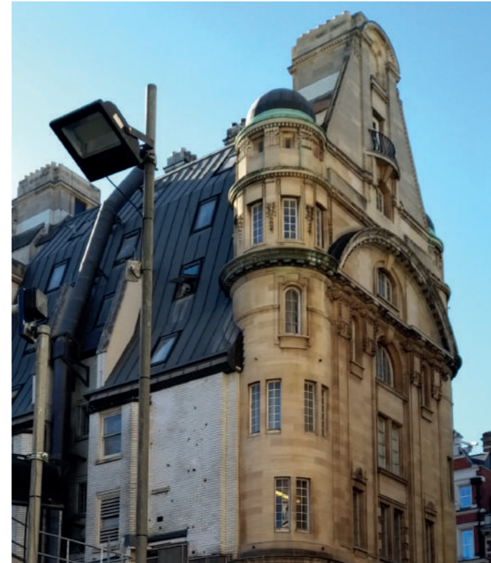
Carlisle House - 'catslide' roof and northern gable
