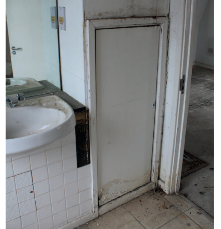
Former upper floor bathroom
