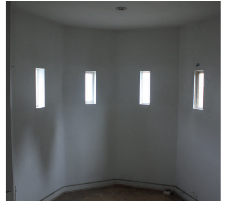
6th floor turret windows & plasterboard lined interior
