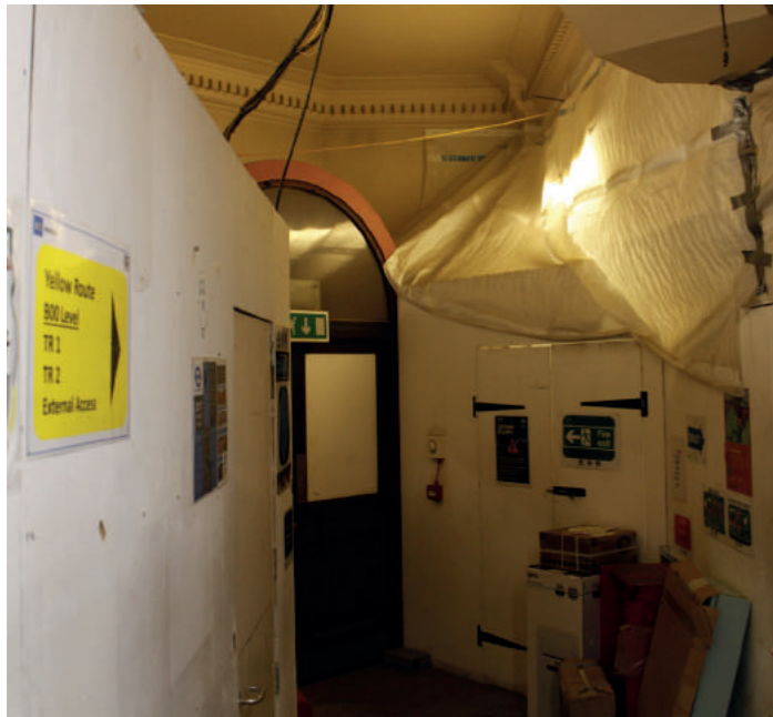
Southwest entrance with Crossrail partitions
