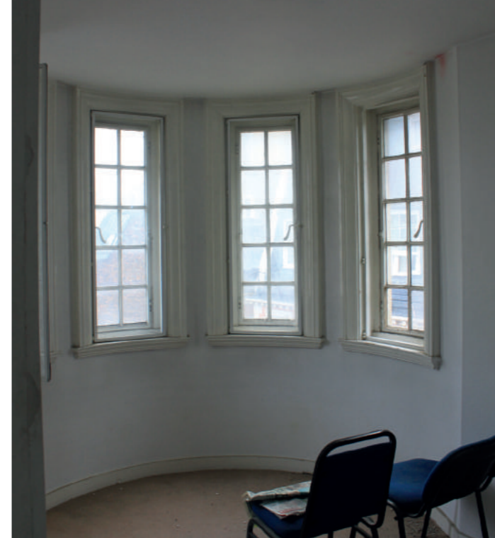
Corner windows and secondary glazing at 1st floor
