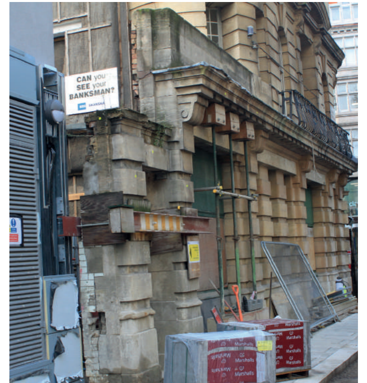
Remaining northern wall of demolished rear extension
