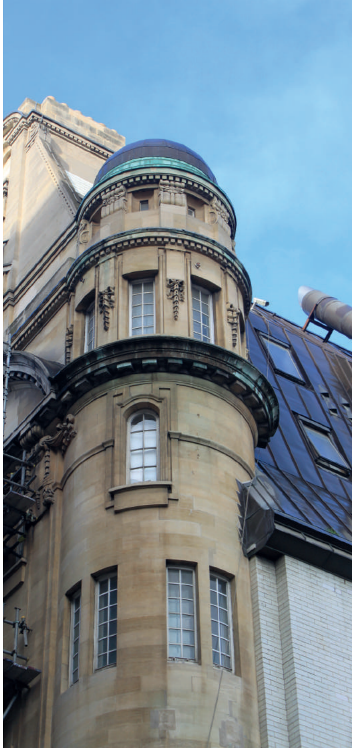
Southeast turret view from Catton Street
