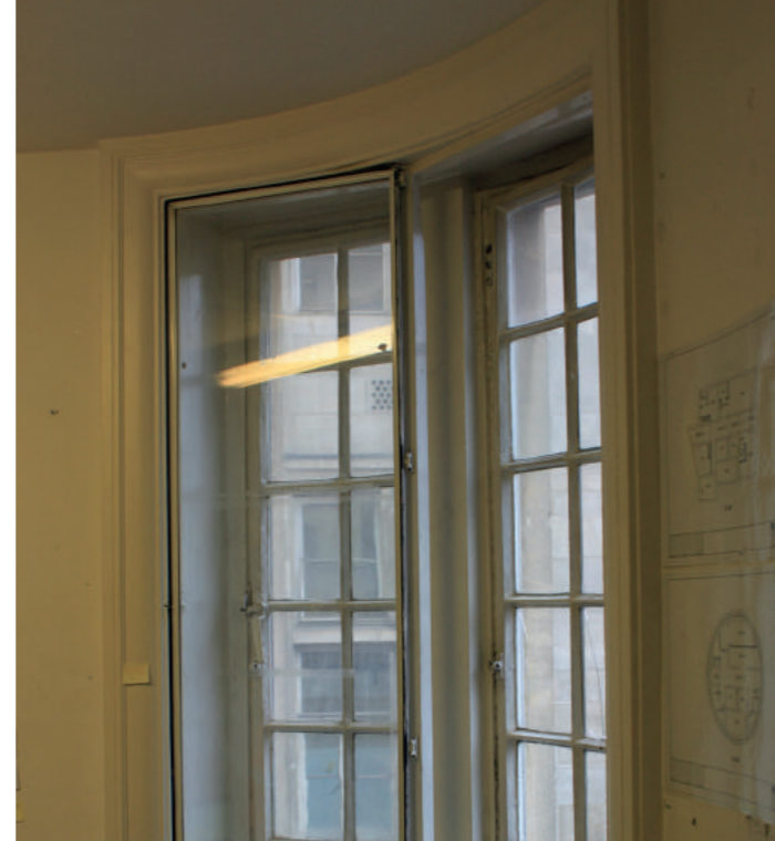
Corner windows and secondary glazing at 2nd floor
