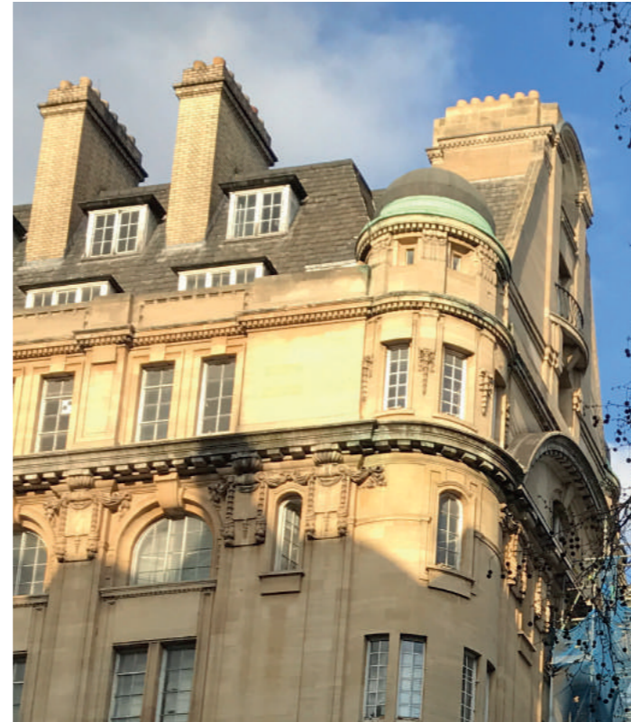
Carlisle House - turrets, chimneys & dormers
