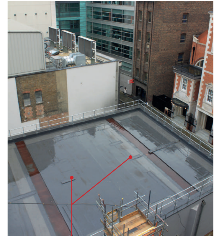
Fixed column positions in TfL headhouse designed to take loading of new building above
