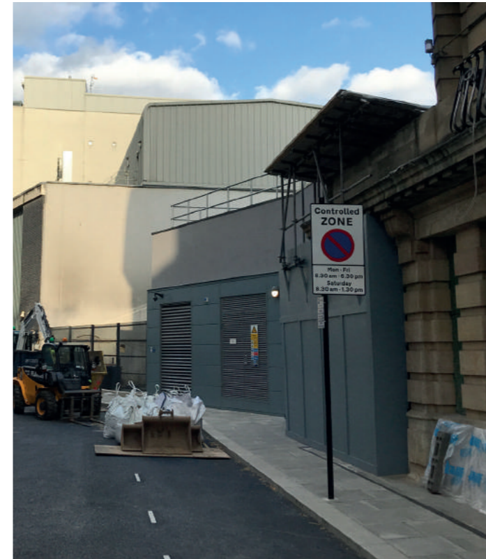
TfL headhouse - Fisher Street looking east
