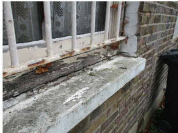
Cracking to cill (note rot to window frame - wear and tear issue)
