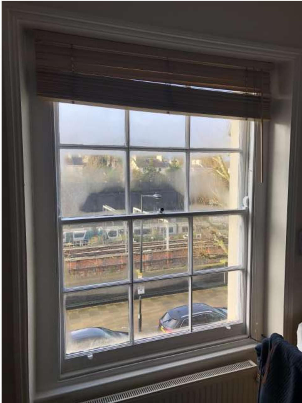
Figure 7: Internal view of the window in the living room at second floor
