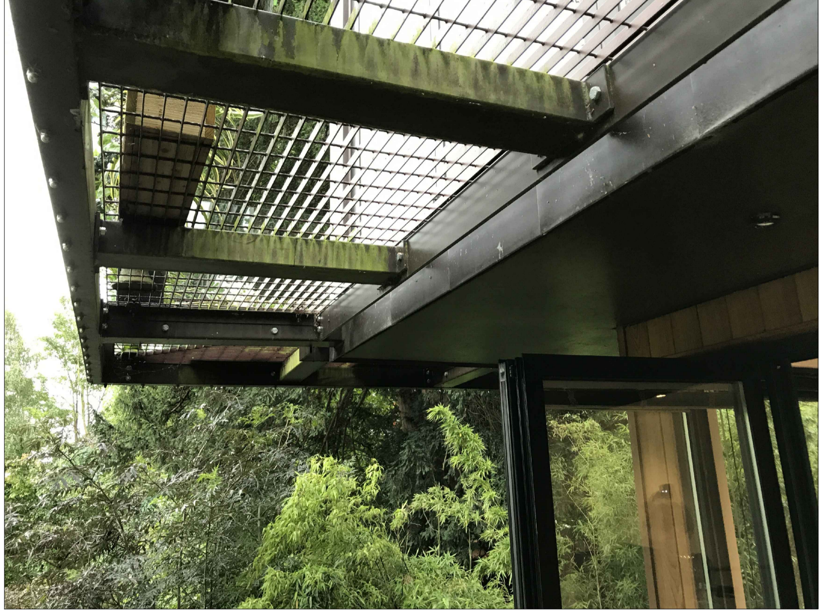
2 Existing First Floor balcony 022 View from existing ground floor terrace
