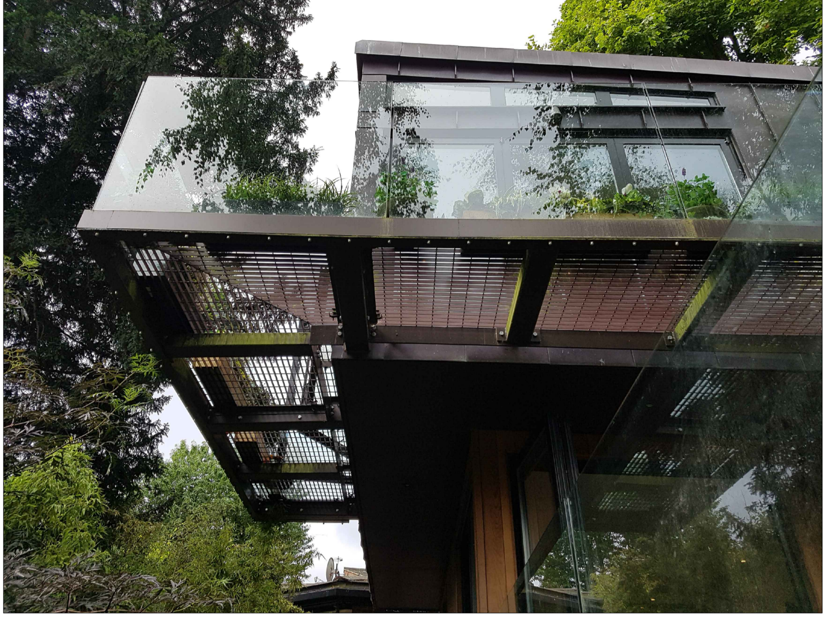
3 Existing First Floor balcony 022 View from existing ground floor terrace
