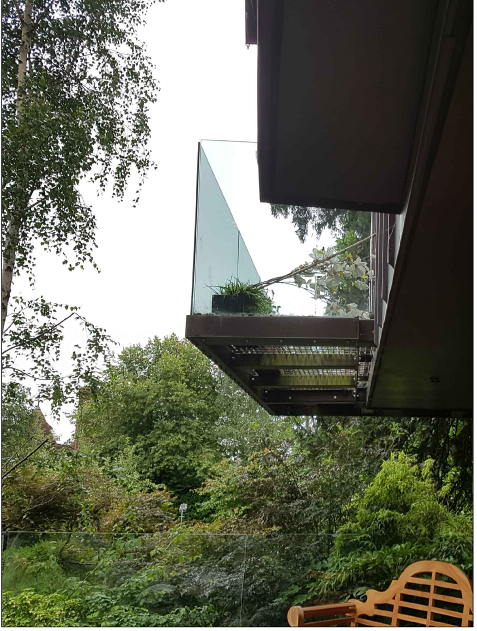
4 Existing First Floor balcony 022 View from existing ground floor terrace
