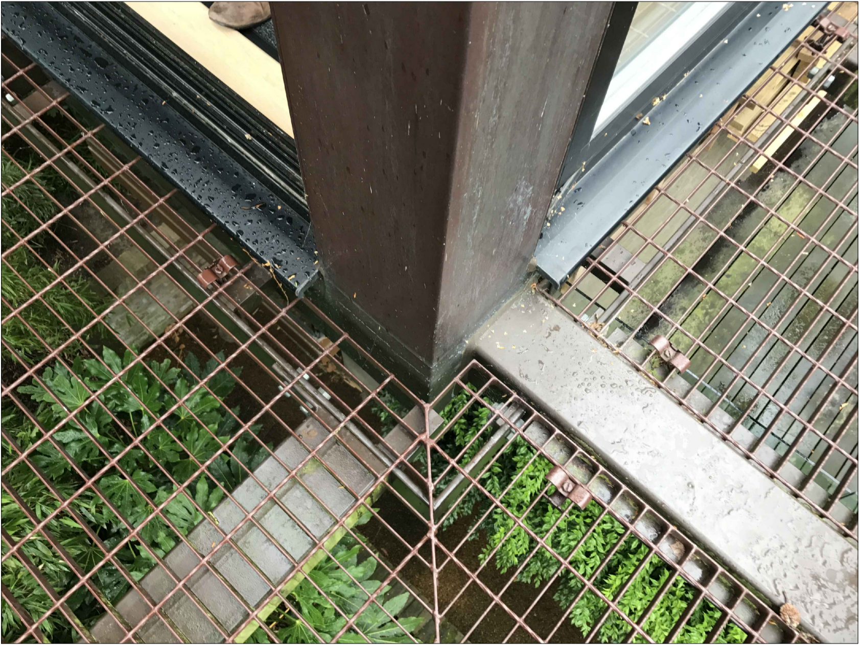
8 Existing First Floor balcony 022 View from balcony
