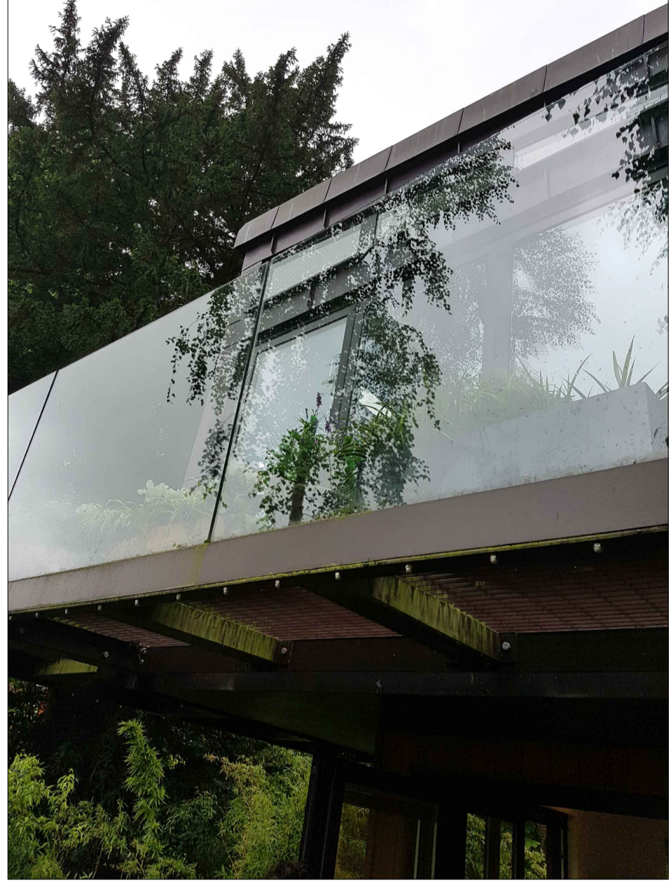
1 Existing First Floor balcony 022 View from existing ground floor terrace
