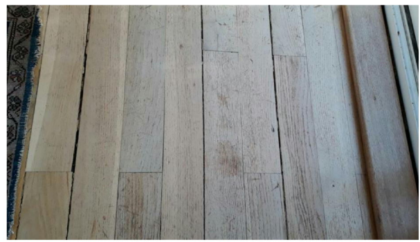
Distorted wooden flooring in rear extension
