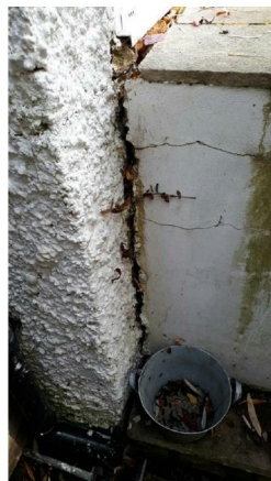
12mm crack where raised patio area pulling away from rear extension
