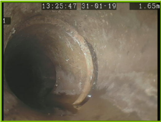
Fig 1.1: Joint displacement on line 1
