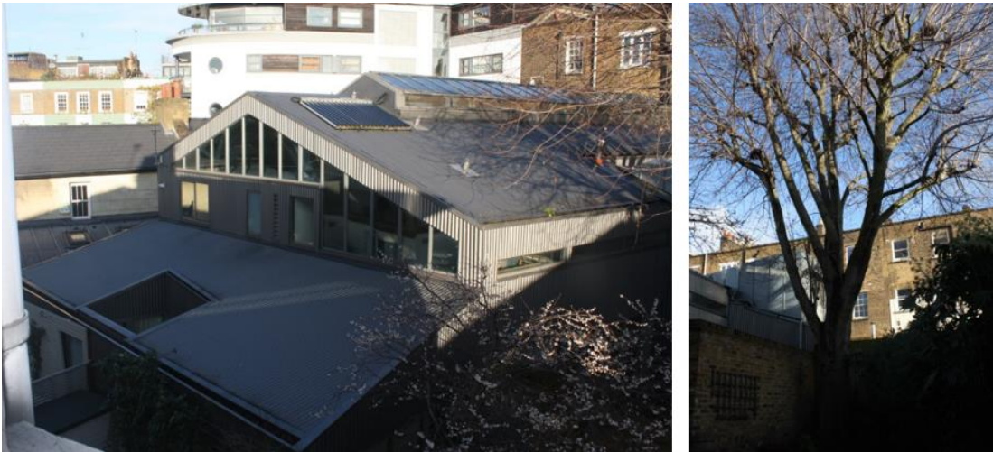
LIVE-WORK BUILDING (LEFT) AND SILVER MAPLE (RIGHT)
