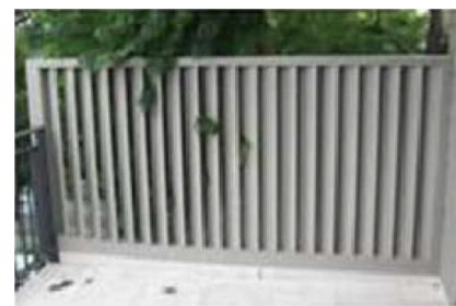
Proposed louvred railings 1200mm height
