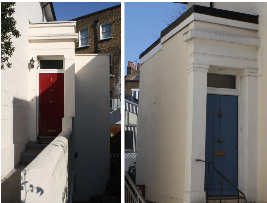
EXISTING TWO-STOREY SIDE EXTENSIONS AT NOS. 1 & 6
