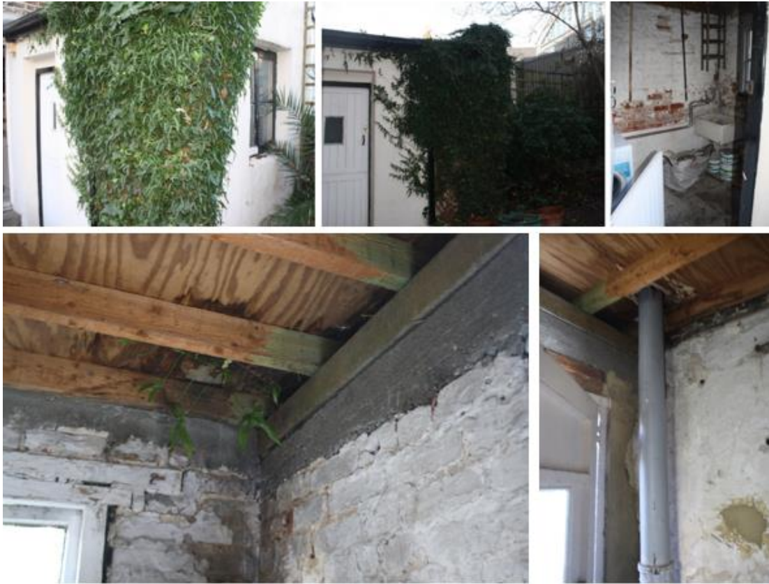
EXISTING REAR EXTENSION
