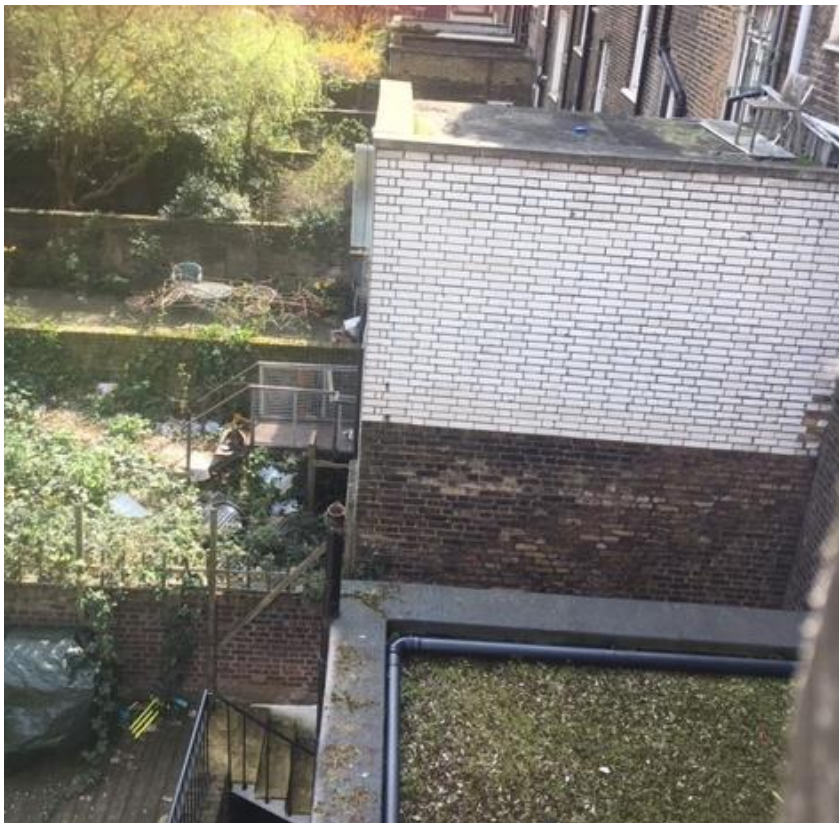
Figure 8 – Closet wing of 23 Harrington Square.
