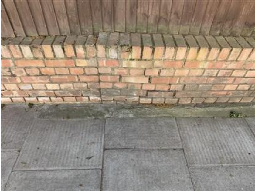
Diagonal cracks (1)
