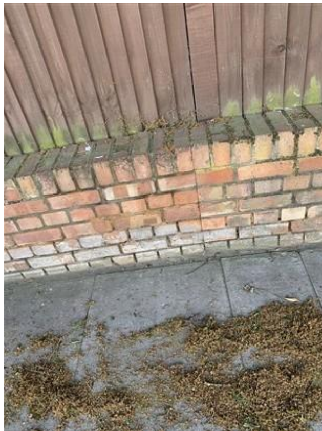
Vertical joint staggered
