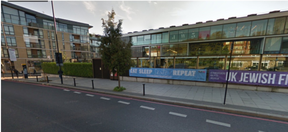
Photo 3 (above): View of neighbouring flats at the Pulse Apartments, 52 Lymington Road
