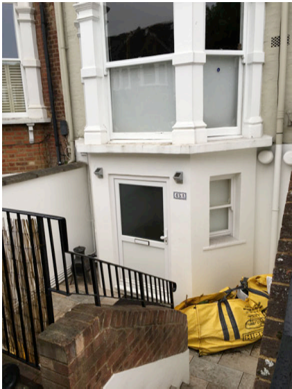
Neighbouring lower ground floor flat at no.45a
