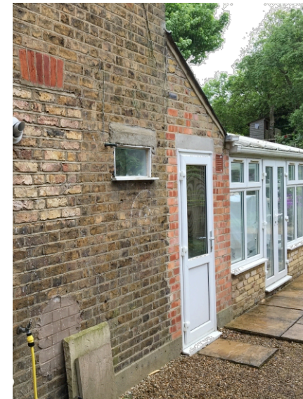
Rear Closet Wing, Porch and Conservatory
