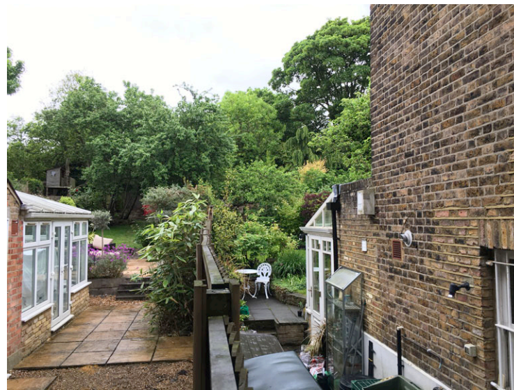
Side return condition w/ no.45
