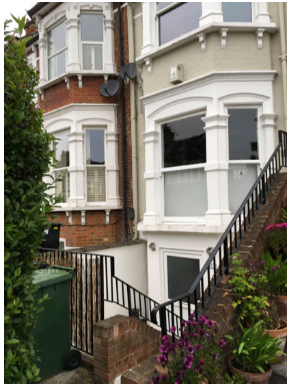
Neighbouring lightwell at no.45a
