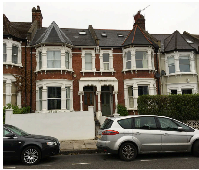
Neighbouring bin store at no.41
