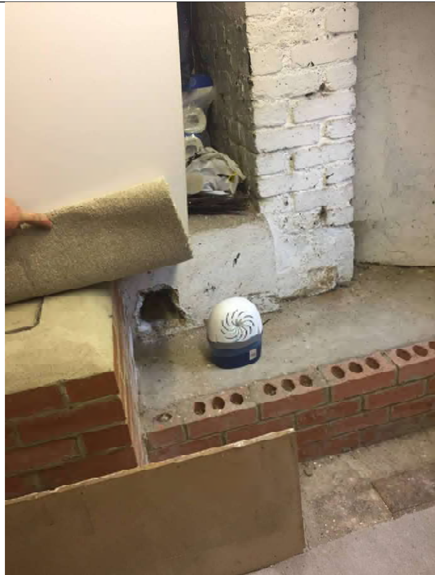
Plate 4: Drain cover within existing basement/cellar.
