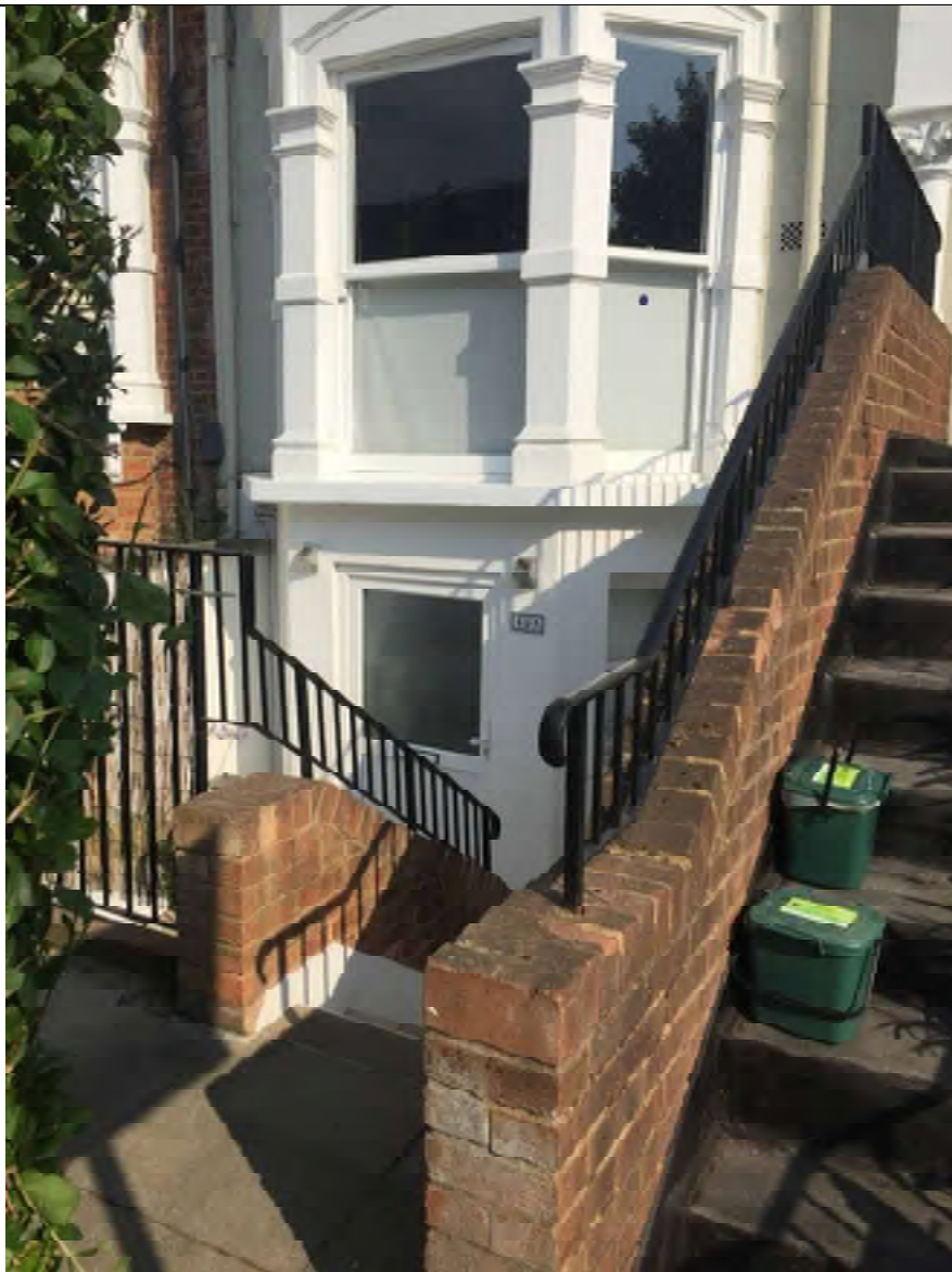
Plate 5: Existing basement in neighbouring property (no. 45).
