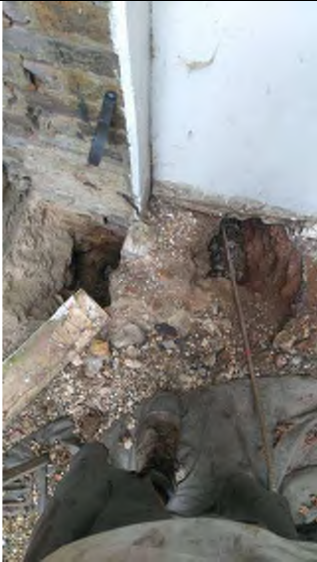
Trial Pit TP1a & 1b
