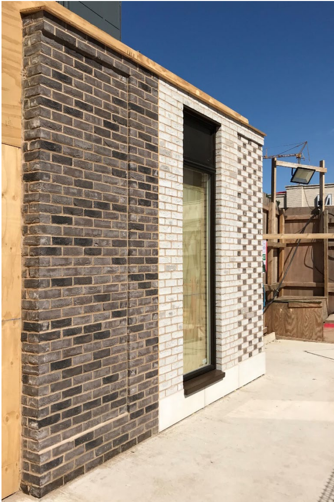
Courtyard Brick & Textured Panels
