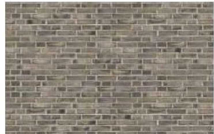
Described in DAS (Vol III , Fig 3.83) as: Stock brick in the 'red-brown-buff range'
