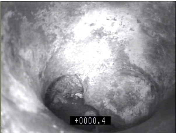
Photo: 6_6a 0.4m, Survey abandoned
