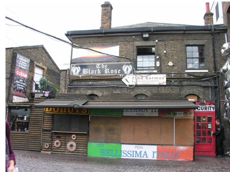
Figure 10 Existing signage within the market
