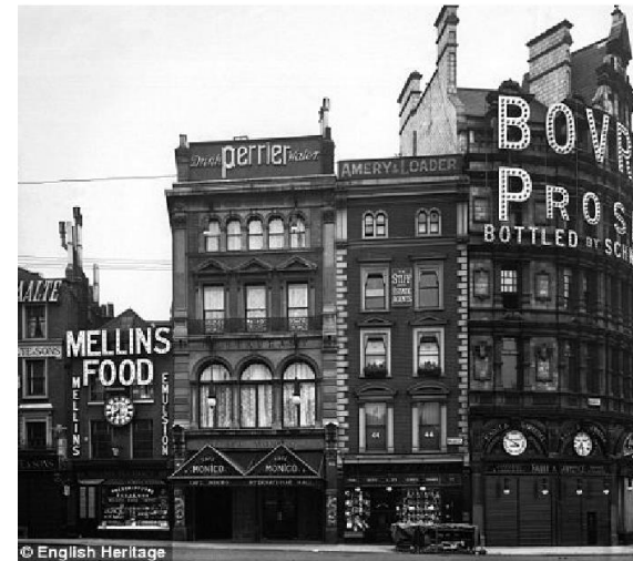
Figure 3 Regent Street in 1910. Source: English Heritage
