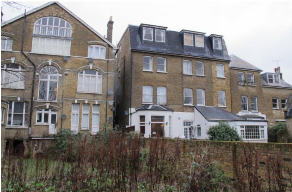
Photo 5 – Rear elevation showing relationship with no.3 Cleve Road
