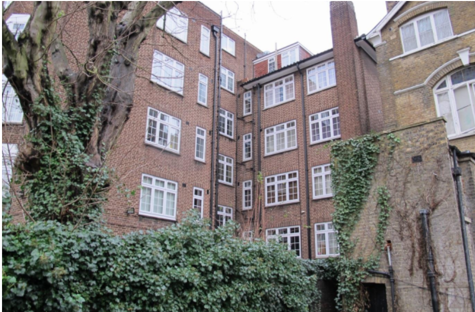
Photo 6 - Rear elevation showing relationship with no.7-9 Cleve Road
