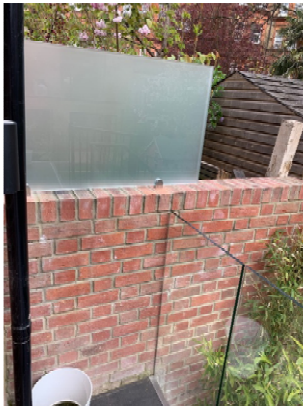
Photo 2 (above): View of privacy screen on boundary with no. 1 King's College Road
