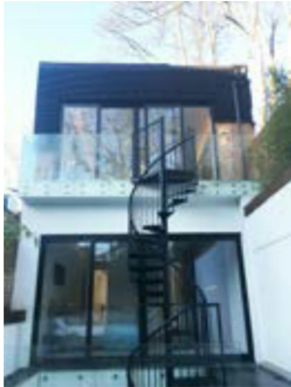
Photo 1 (above): View of rear ground and upper ground floors with installed staircase
