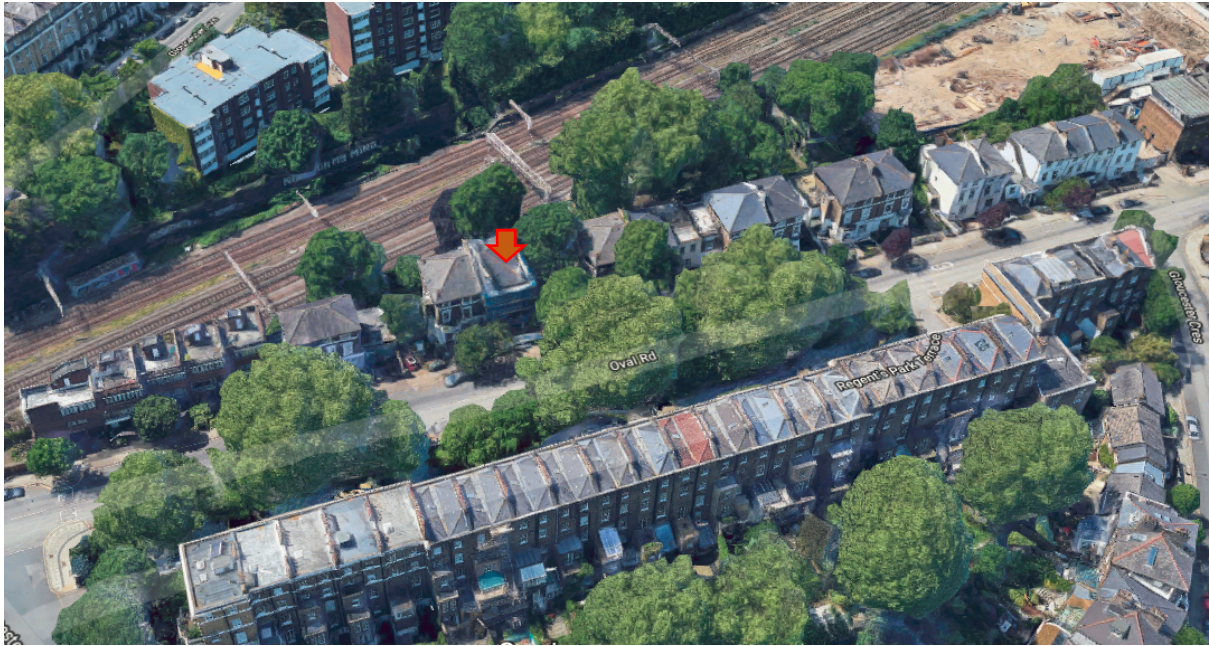
Photo 1 (above): Aerial view of 5 Oval Road
