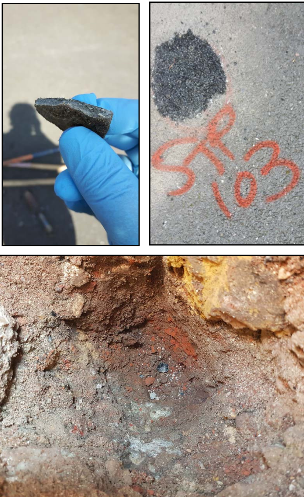
Figure 3. Excavation, reinstatement and Asbestos Cement Board identified in STP103.
