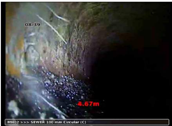
, 00:01:04, 4.67 m Roots, fine at joint
