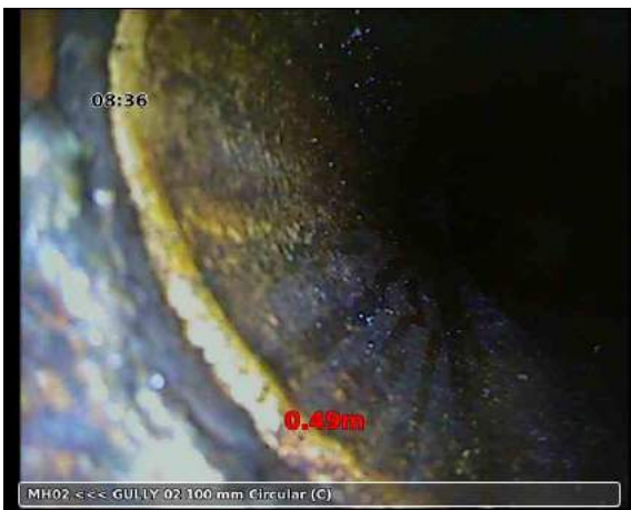
, 00:00:29, 0.49 m Survey abandoned, UNABLE TO PUSH UP
