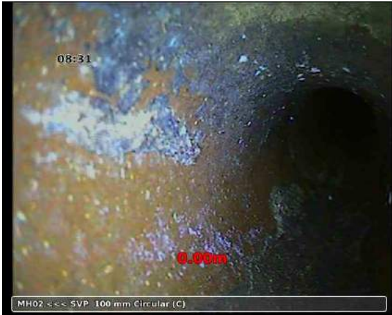
, 00:00:05, 0.00 m Start node type, manhole, reference number: MH02
