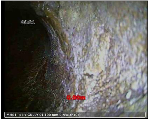
, 00:00:03, 0.00 m Start node type, manhole
