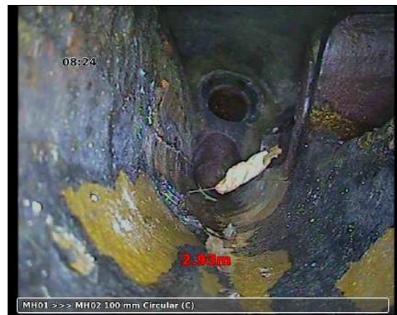
, 00:00:57, 2.93 m Finish node type, manhole, reference number: MH02
