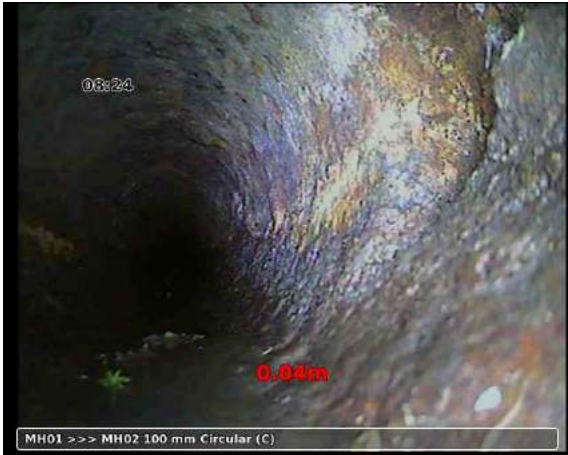
, 00:00:18, 0.04 m Start node type, manhole, reference number: MH01
