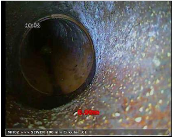
, 00:00:06, 0.00 m Start node type, manhole, reference number: MH02
