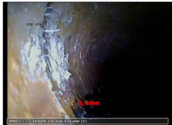
, 00:01:08, 5.40 m Roots, fine at joint
