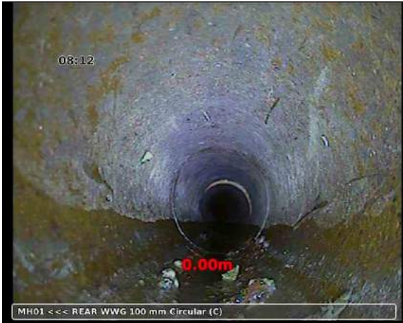
, 00:00:04, 0.00 m Start node type, manhole, reference number: MH01
