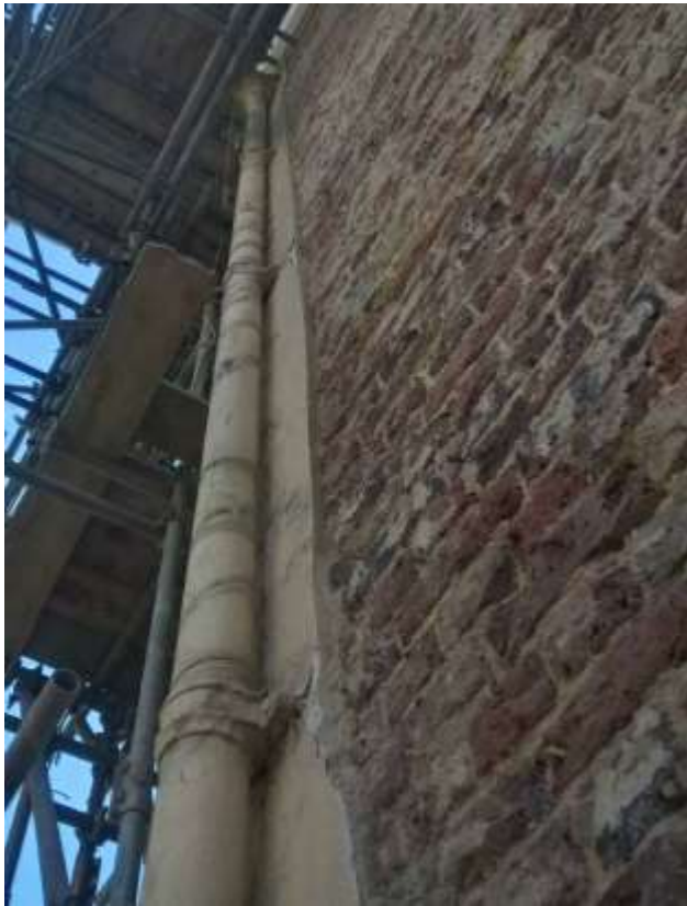
Above: modern 'Timesaver' rainwater pipe proposed for removal (item 13)
