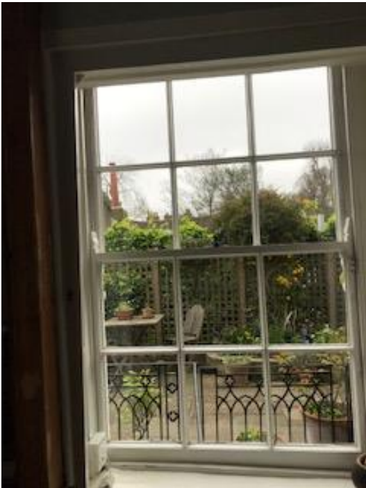
Item 2 - Ground floor Front Elevation Living Room Sash window
