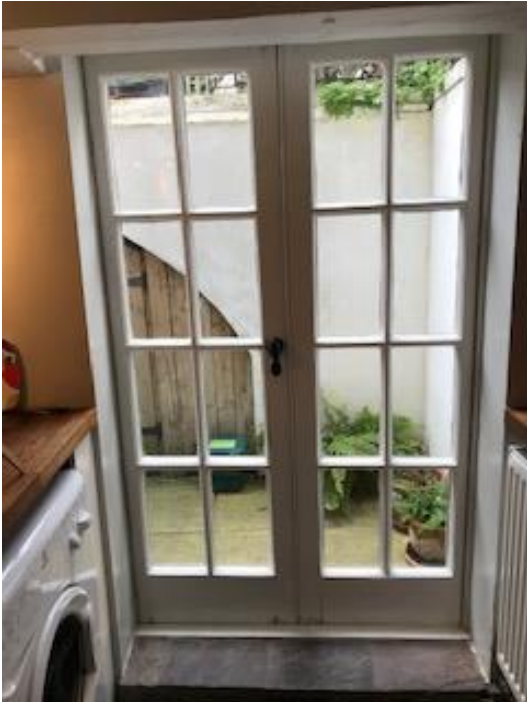
Item 1 - Kitchen basement front elevation French Windows/door
