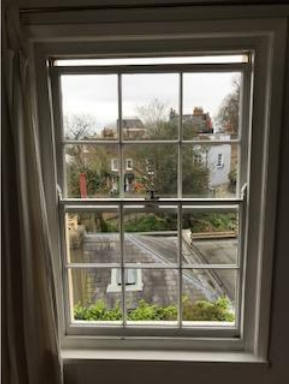
Item 6 - 2nd floor front elevation bedroom sash window
