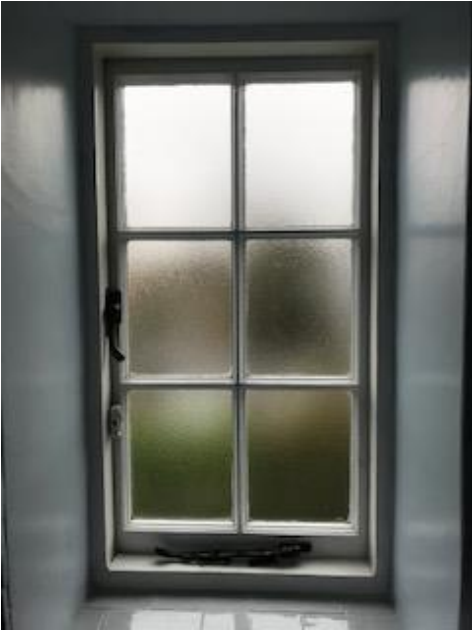
Item 4 - 1st floor Front Elevation Bathroom Casement window
