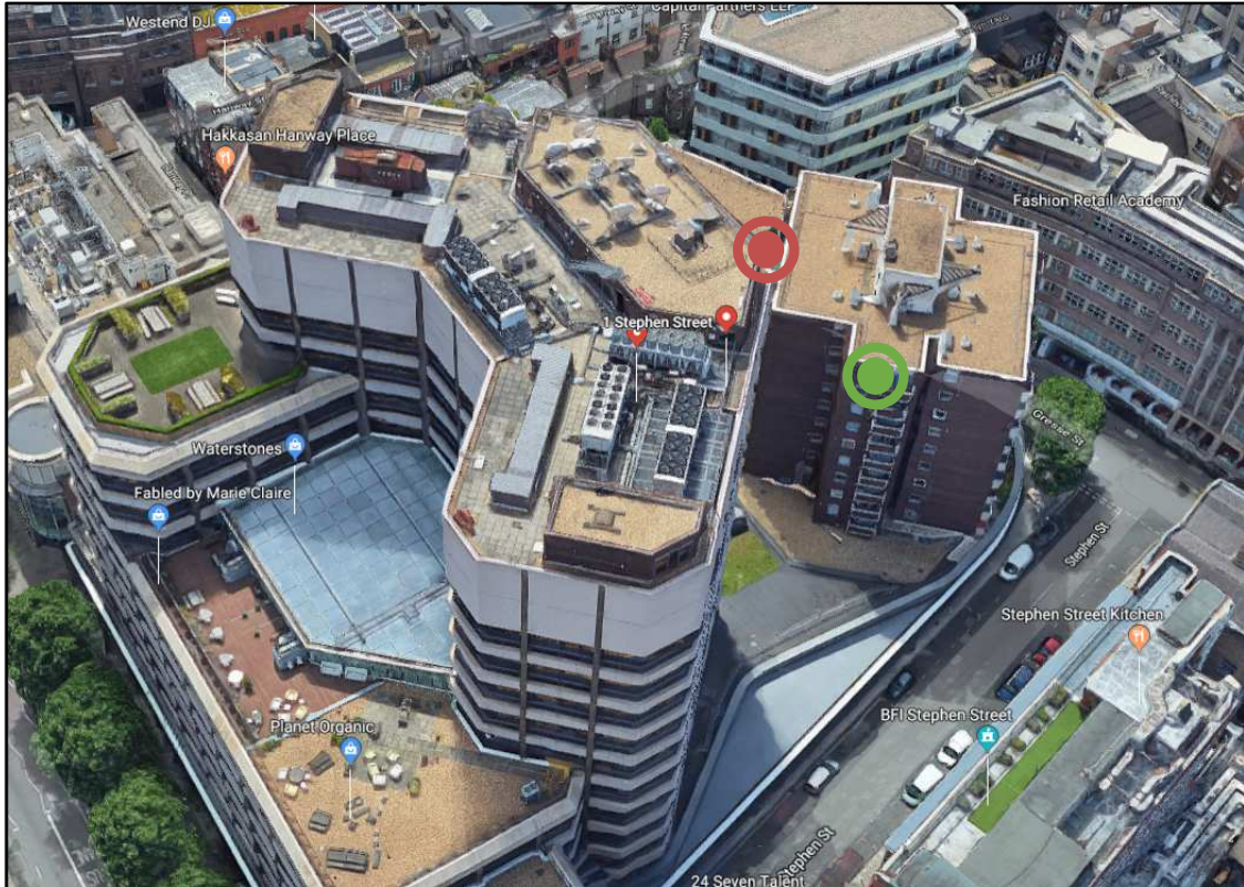
Figure 2.3 Site measurement position and identified closest noise sensitive receiver (Image Source: Google Maps)
