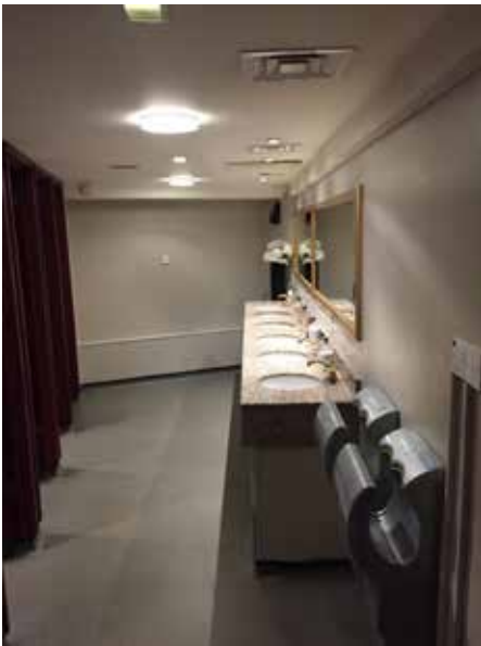
Fig 2. Existing Vanity Unit
