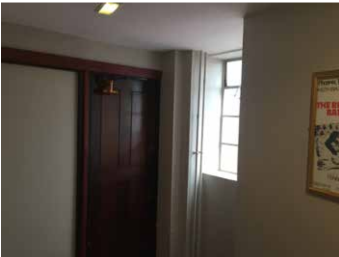
Fig 5. Existing Door To Washroom
