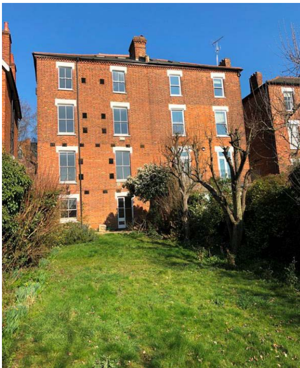
Rear elevation of No. 9 & No. 11 Nassington Road
