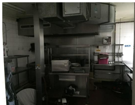
Figure 8: Kitchen at second floor
