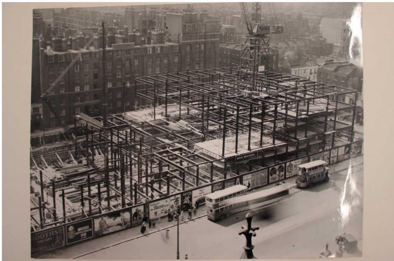
Figure 3.6 Photo taken during construction of steel frame
