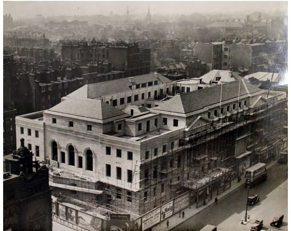
View from the north-east of the Euston Road with Queen Alexandra Mansions in the background showing the near completion of the building (the roof pavilions had been completed since the last image and most of the scaffolding removed from the eastern elevation), March 14, 1936 (© Camden Local Studies: 31.801, DIG 06057)
