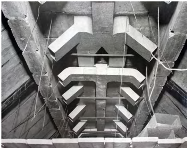
Air ducts fitted into the roof of the Council Chamber, March 1936 (© Camden Local Studies: LCP 725.13, D. M. Wolfe, NEG 148)
