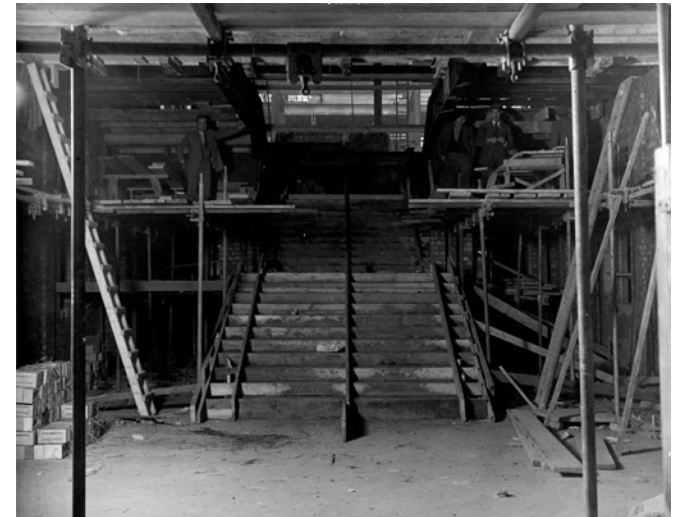
Staircase in the Entrance Hall under construction, November 27, 1935 (© Tim Drewitt)
