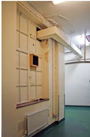
The south-west lightwell has been infilled but its volume and windows remain
