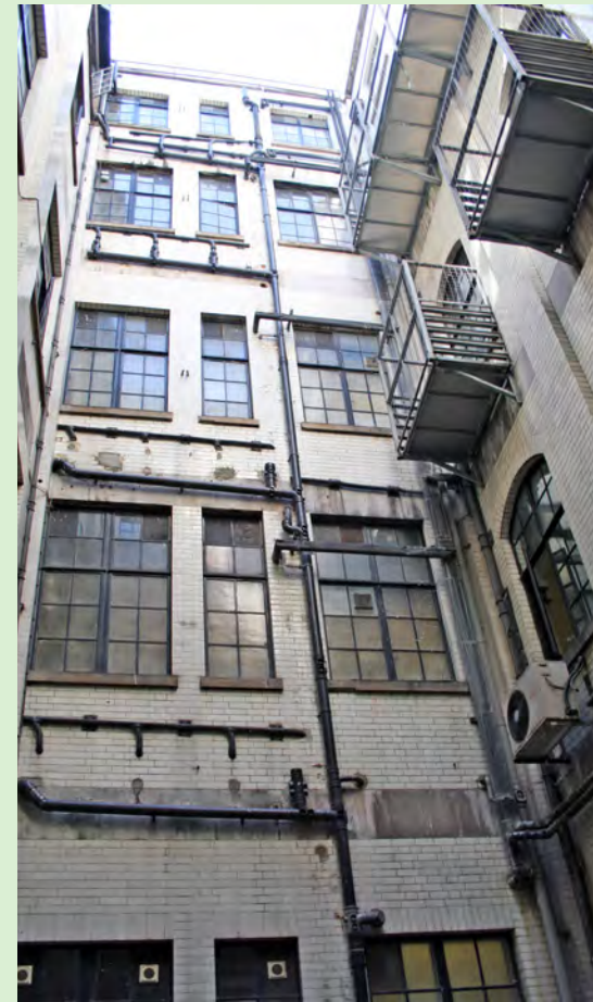
Waste pipes on the north-west lightwell, note the air-conditioning units in cages to the right. The lightwells are clad with white glazed tiles.
