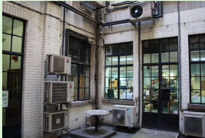
Air-conditioning units, pipework and cabling attached to the tiled walls of the north-west lightwell
