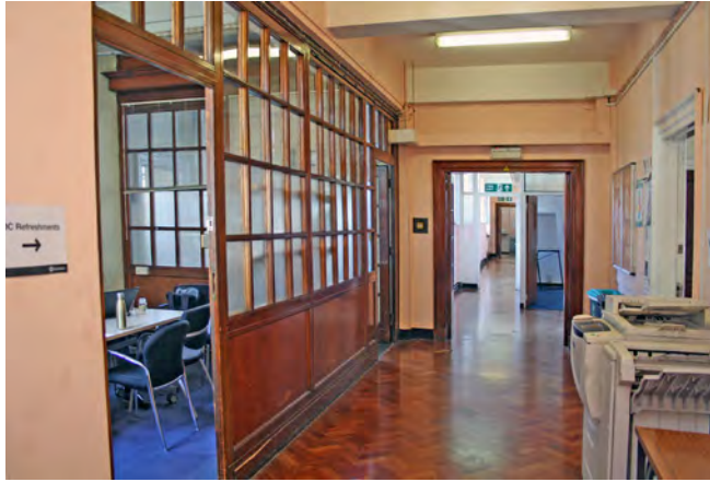
Southern part of encircling corridor with non-original timber and glazed partition to left side
