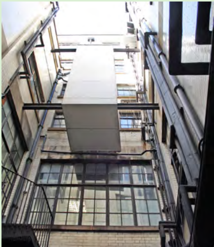
The north-east lightwell has further plant and a platform lift extending between First and Mezzanine floor levels
