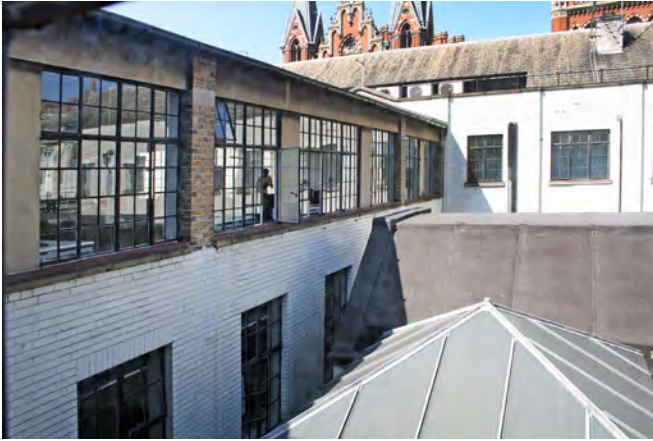
Later extension at Third floor, indicated by the brick finish compared to the glazed tiles below
