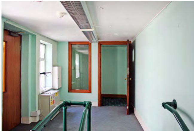
Altered corridor adjacent to northern Mezzanine gallery to allow wheelchair access; the platform lift is through the door on the left.
