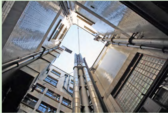
The south-east lightwell contains many exhaust chimneys and other plant
