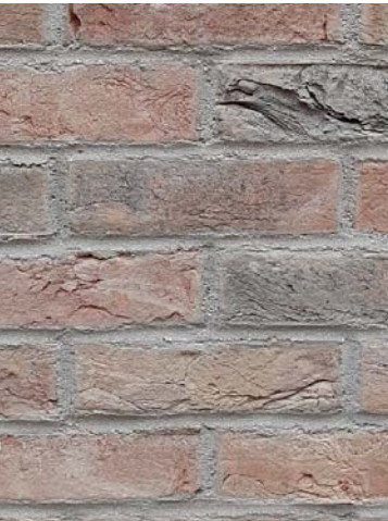
Brickwork mortar - bucket handle joint
