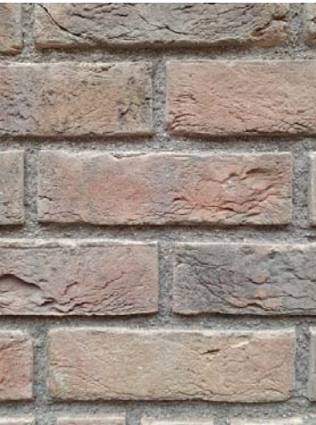
1.2 Brickwork mortar - recessed joint
